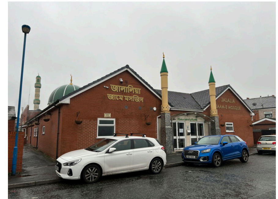
Existing Nile Street View
