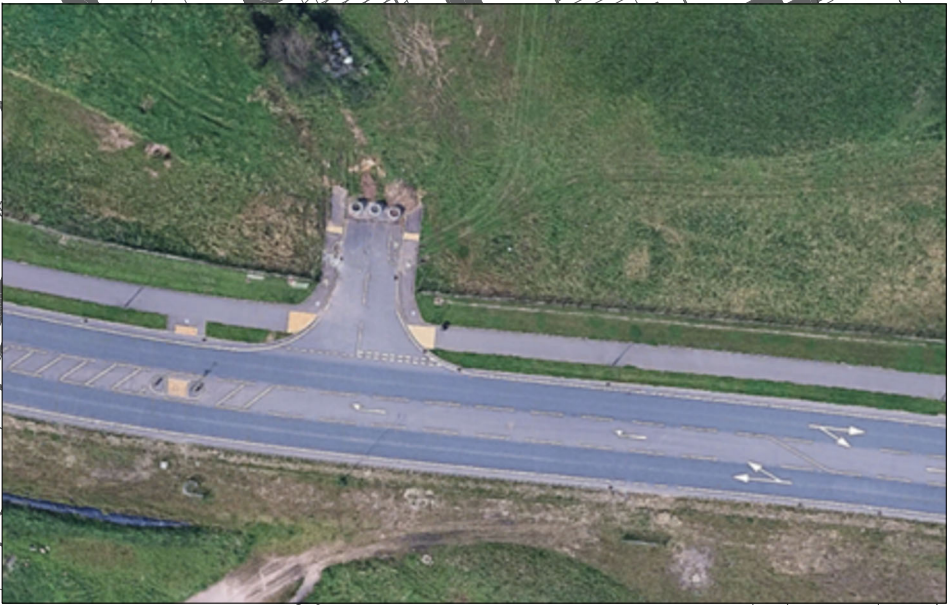
NORTH-SOUTH AERIAL VIEW
