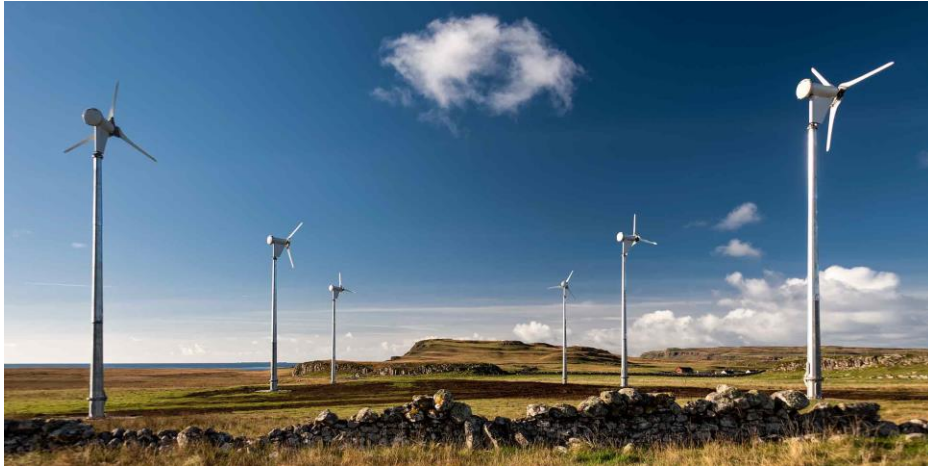
Figure 10: Typical Small Scale 6kW Wind Turbine
