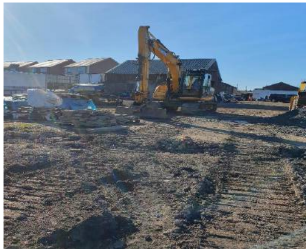
Photograph 2: Machinery storage and containers (TN1)
