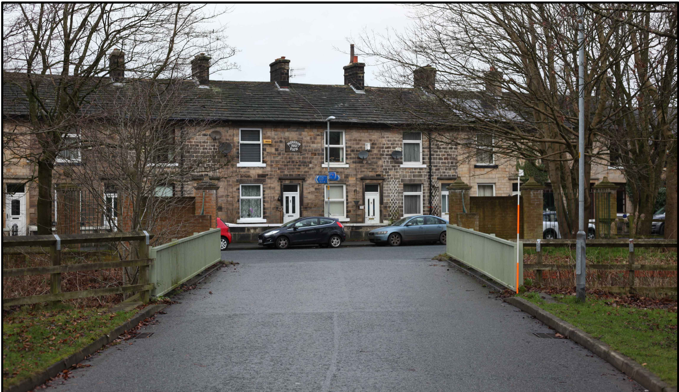
View from the South East
