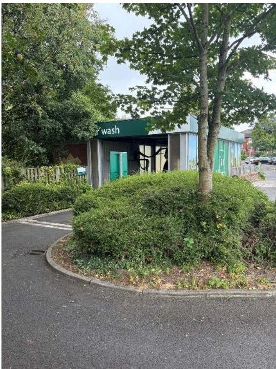
Photograph 6: Building 3 with no bat roost potential.
