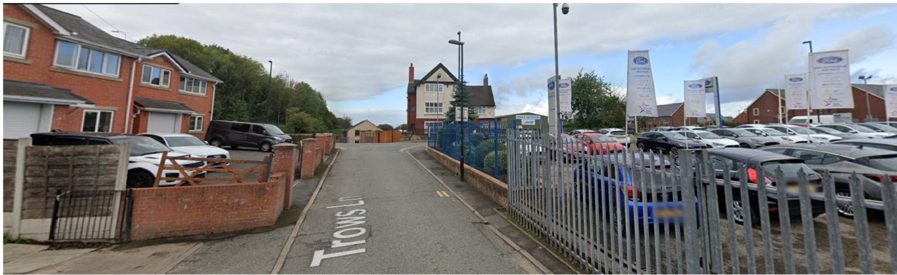
2 Trows Lane (facing West)
