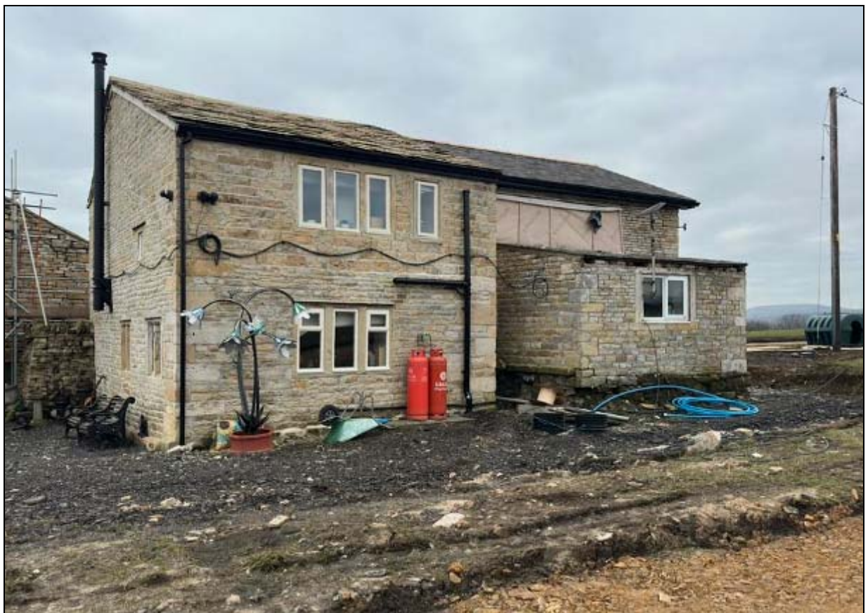
Rear, showing single-storey outshut, again probably later
