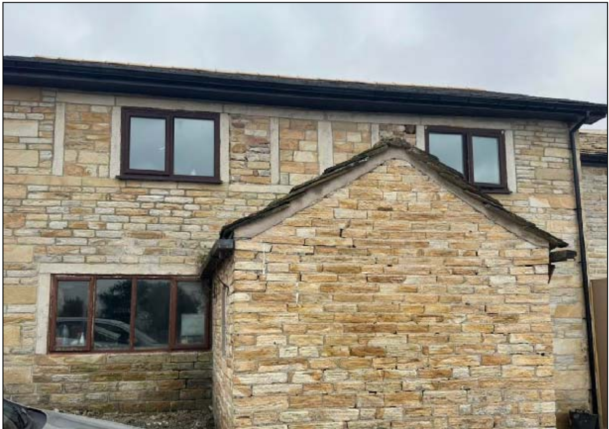
The first floor weavers' window was originally full-length
