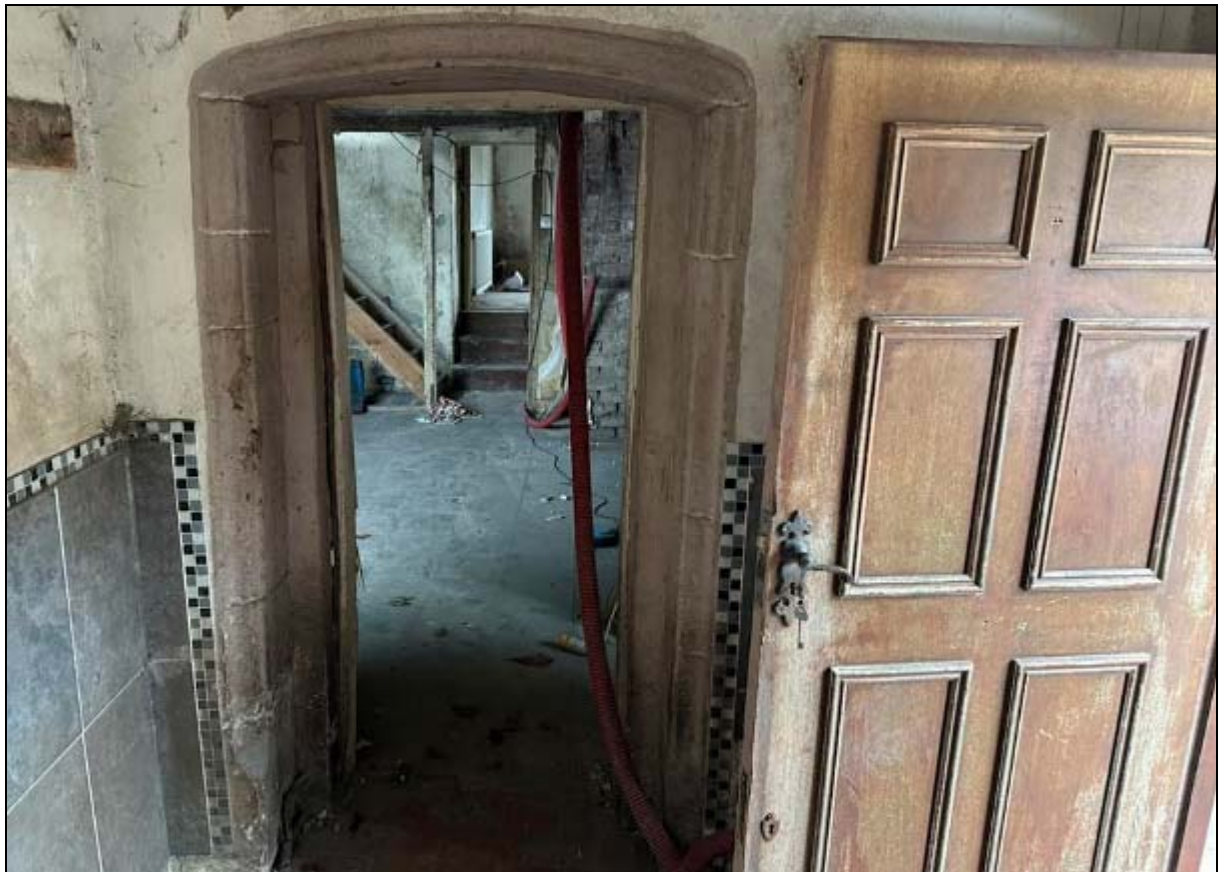
Late 17 th century door surround concealed by the porch
