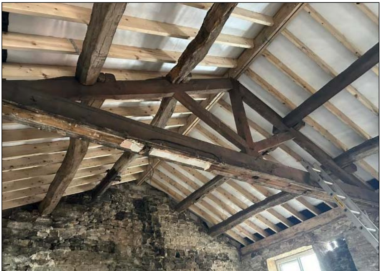
The machine-cut roof truss in the main block confirms an early 19 th century rebuilding date
