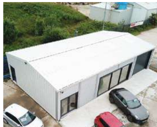
Hanson Industrial Buildings Pages 30-31
