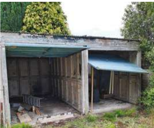
Hanson Garage Refurbs Pages 26-27
