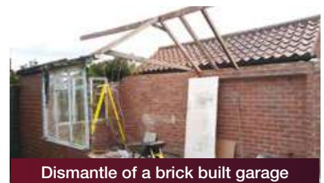
Old damaged roof being replaced
