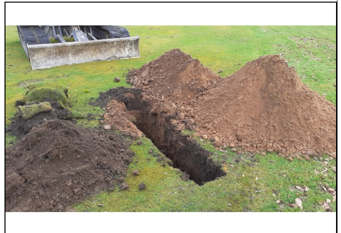
Trial Pit 102 Spoil
