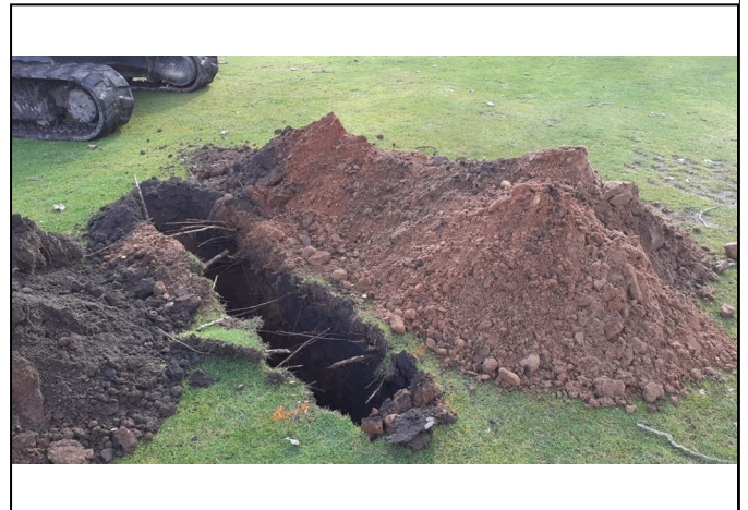
Trial Pit 111/ Soakaway 103 Spoil
