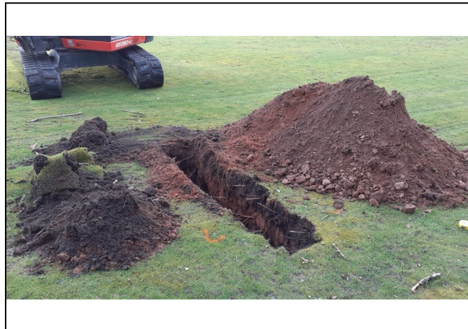
Trial Pit 101 Spoil
