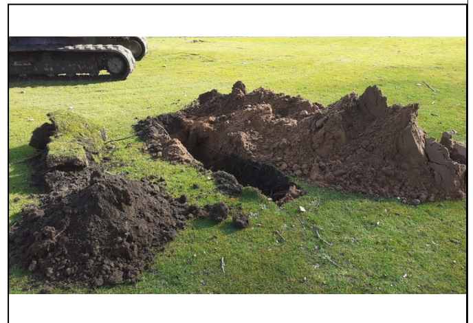
Trial Pit 108 Spoil
