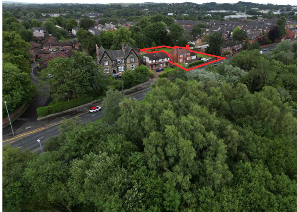
Drone view looking South towards the site
