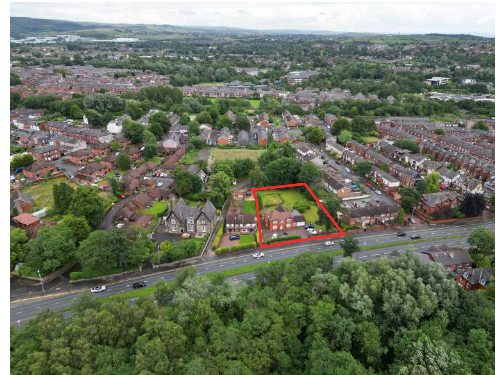
Drone view looking South East towards the site
