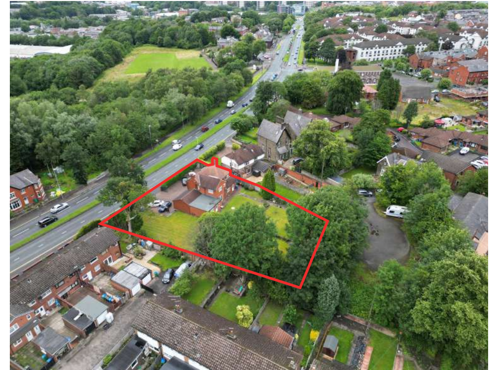
Drone view looking North towards the site
