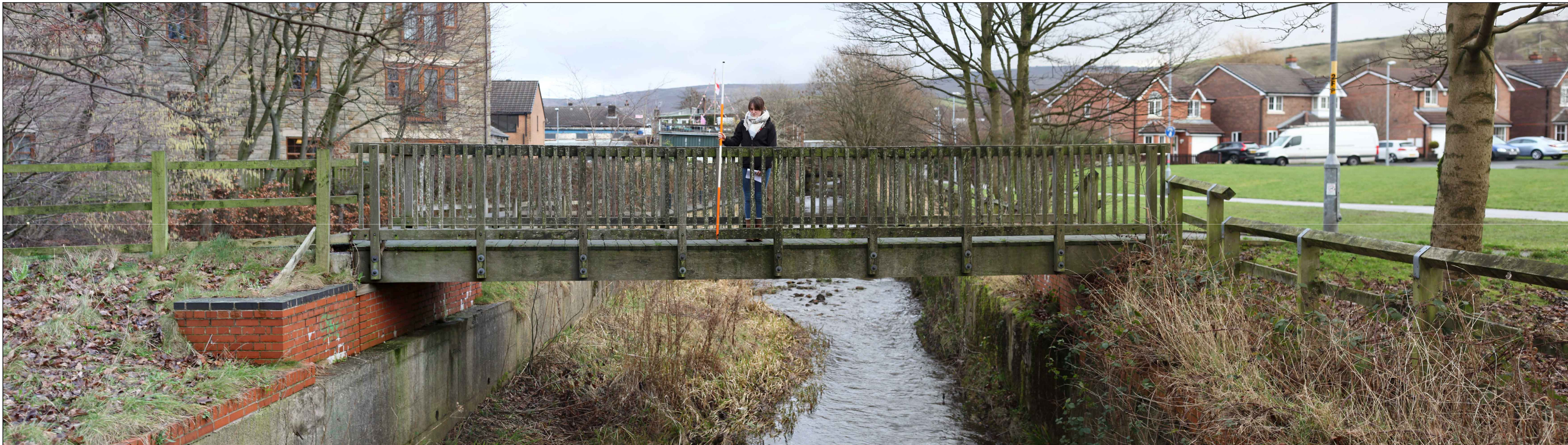
View from the West
