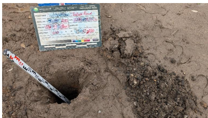
VP4: Overview of Excavation.
