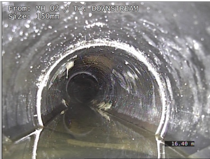
Fracture multiple from 3 to 10 o'clock - Remark: TIMES VARY , Finished
