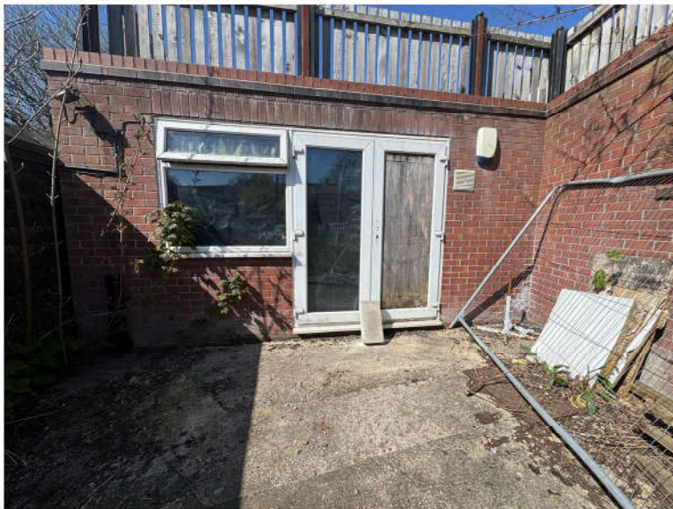
Looking northwest at lower ground floor room
