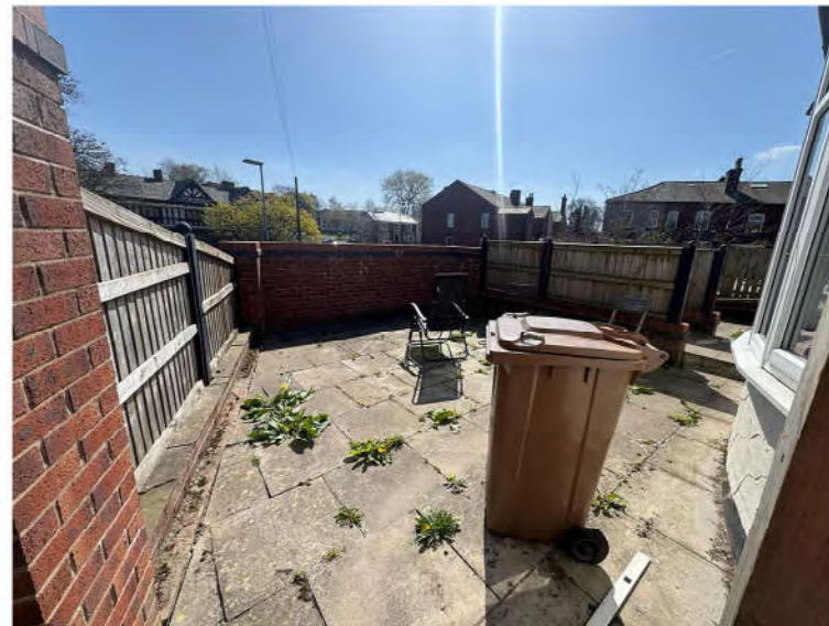
Looking southwest at rear (southwest) corner
