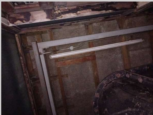
Photograph 7: Water tank room on the roof of Block B.
