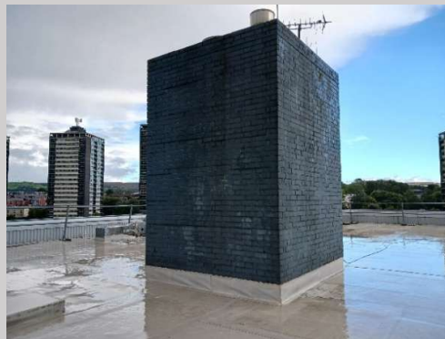
Photograph 8: Brick structure on the roof of Block B. Only accessible externally.
