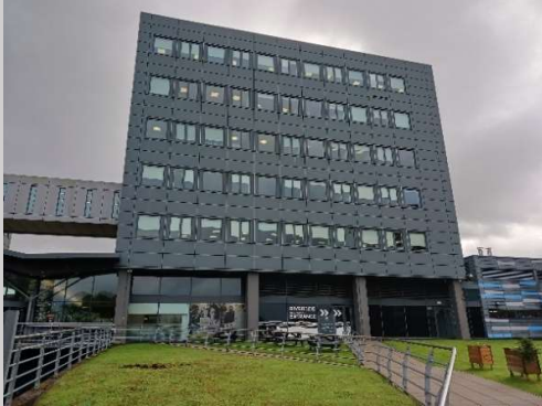
Photograph 1: Block A, connected to Block B.
