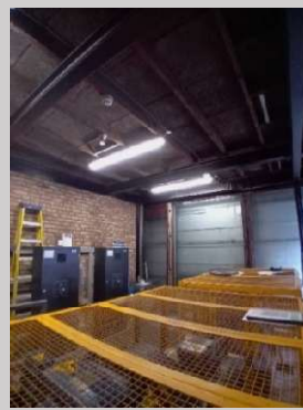
Photograph 6: Interior of roof wiring room, Block B.
