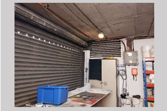
Photograph 15: Internal view of one of the garages. The garages had potential access points for bats.
