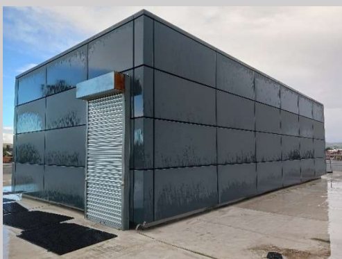
Photograph 11: Metal clad buildings on top of the Block B flat roof.
