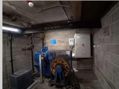
Photograph 4: Winch lift room on the roof of Block A.
