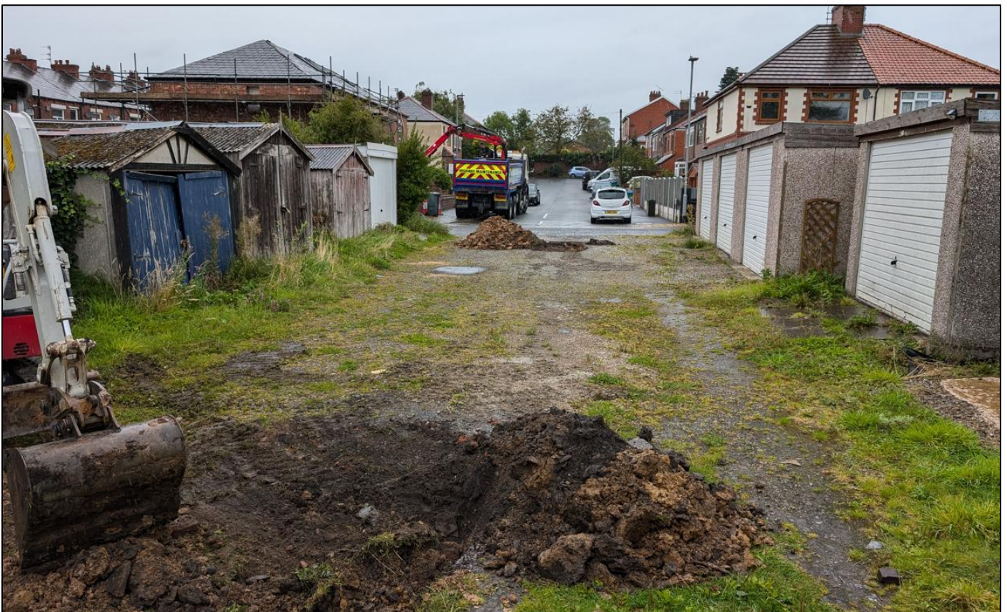
General site photographs.
