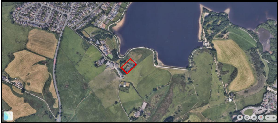
Figure 1: The building location in its wider setting (shown with red keyline).
