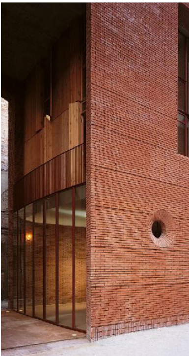
Red facing brickwork pattern and timber windows
