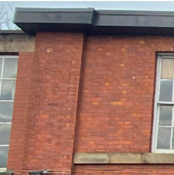
Red Facing Brickwork
