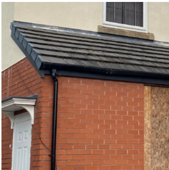
Pitched Roof of Side Extension
