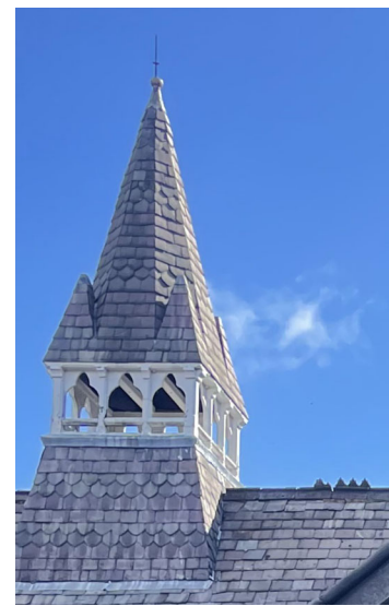
Cupola tiling intact
