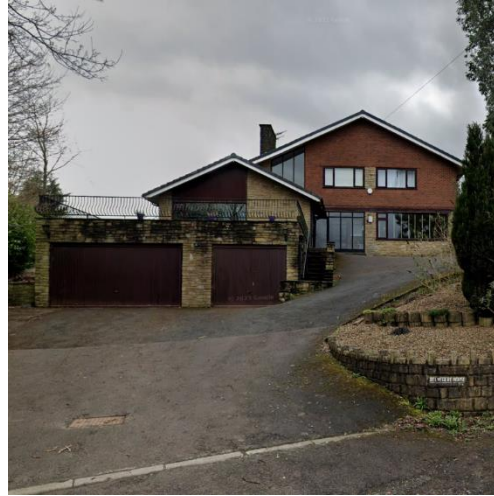
2. Stone, red brick and cladding houses.
