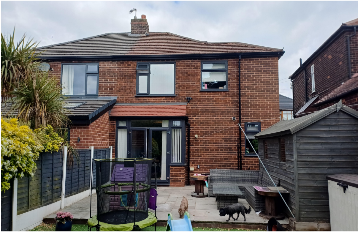
View to rear of property
