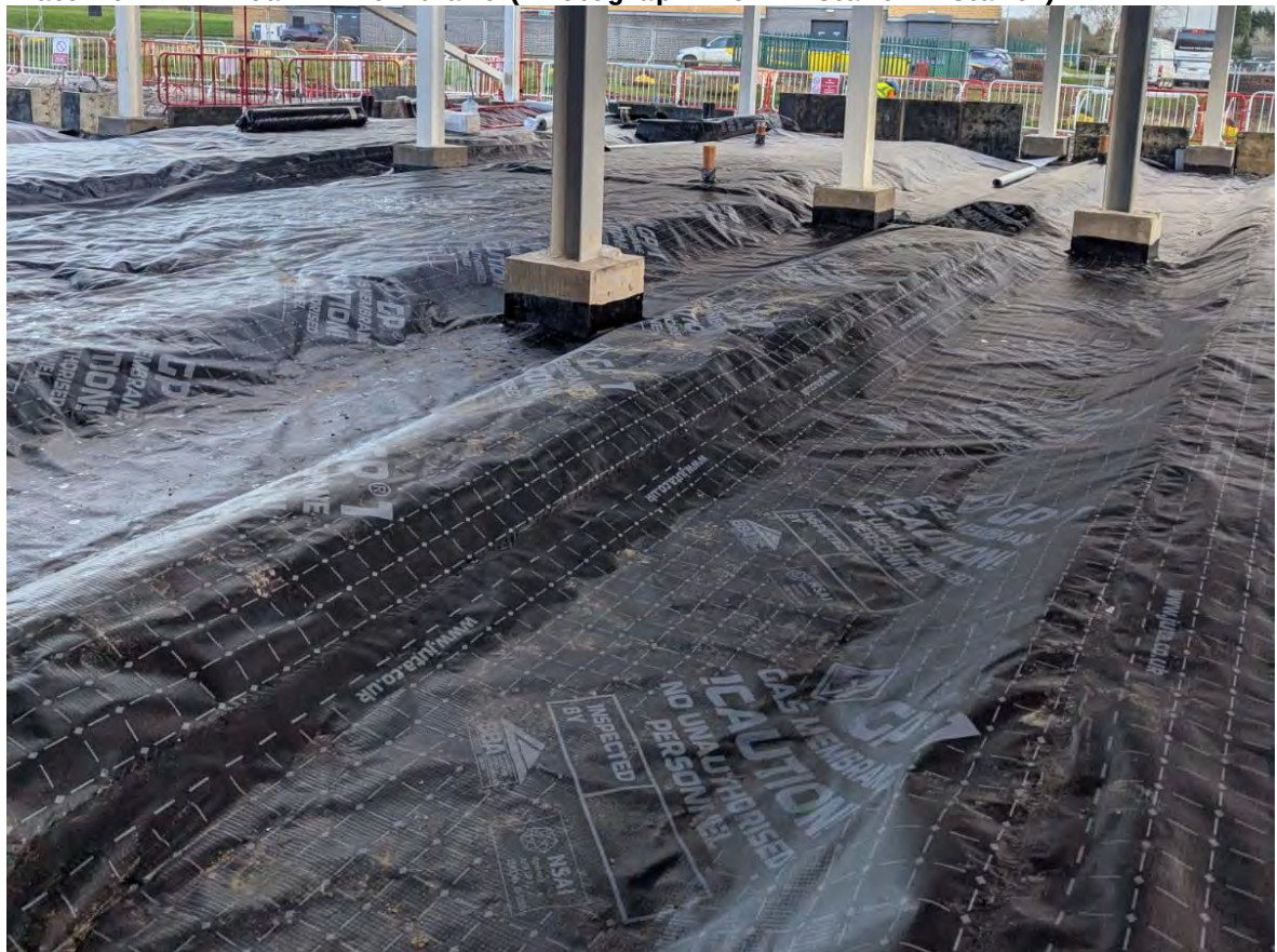
Plate 26 Area 1 – Membrane (Photograph From Installer Installer)
