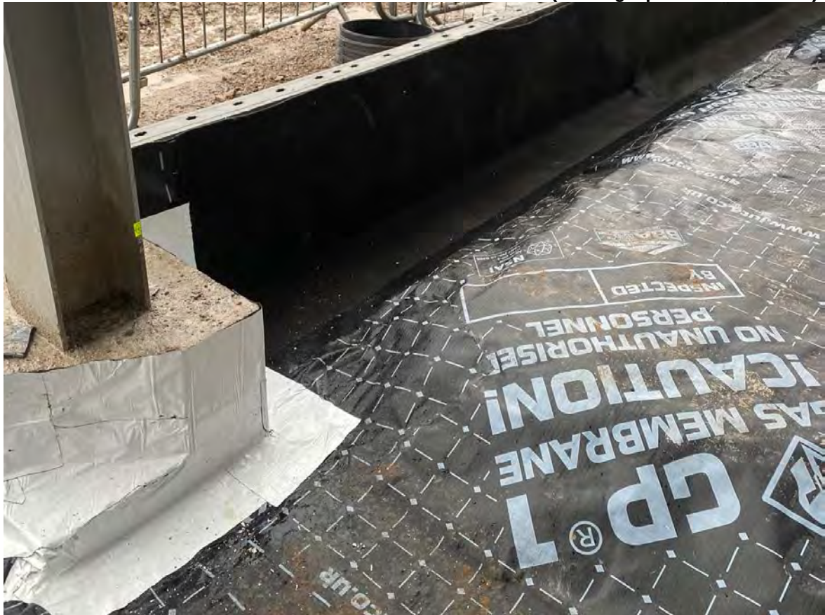
Plate 34 Area 3 – Perimeter and Sealed Penetration (Photograph From Installer)
