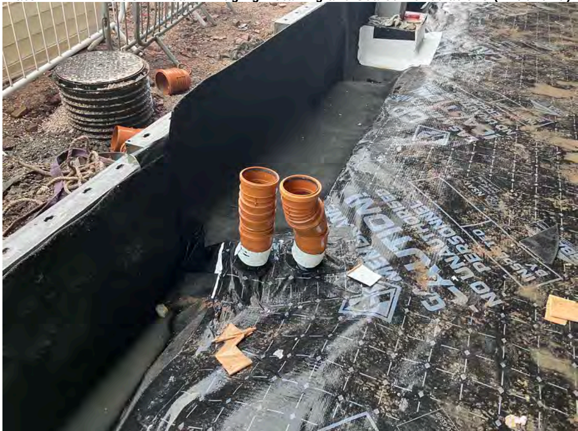
Plate 12 Visit 3 – Area 2 – Edging Detailing and Sealed Penetrations (14/01/25)
