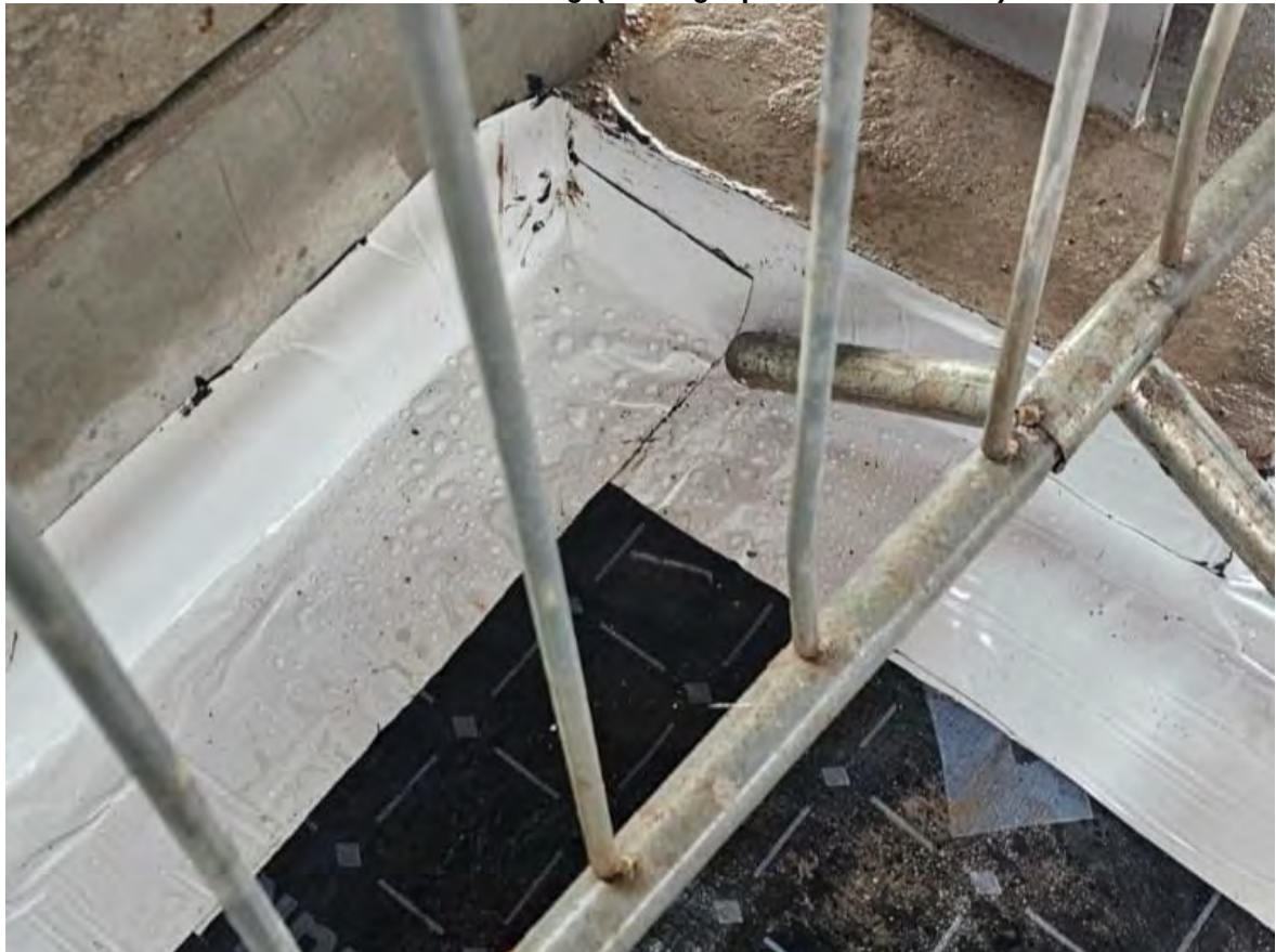
Plate 30 Area 2 – Corner Detailing (Photograph From Installer)
