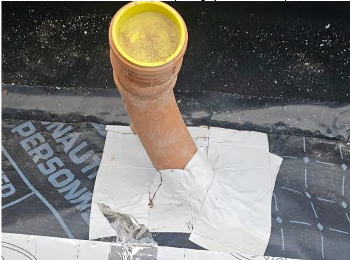
Plate 28 Area 1 – Sealed Penetration (Photograph From Installer)
