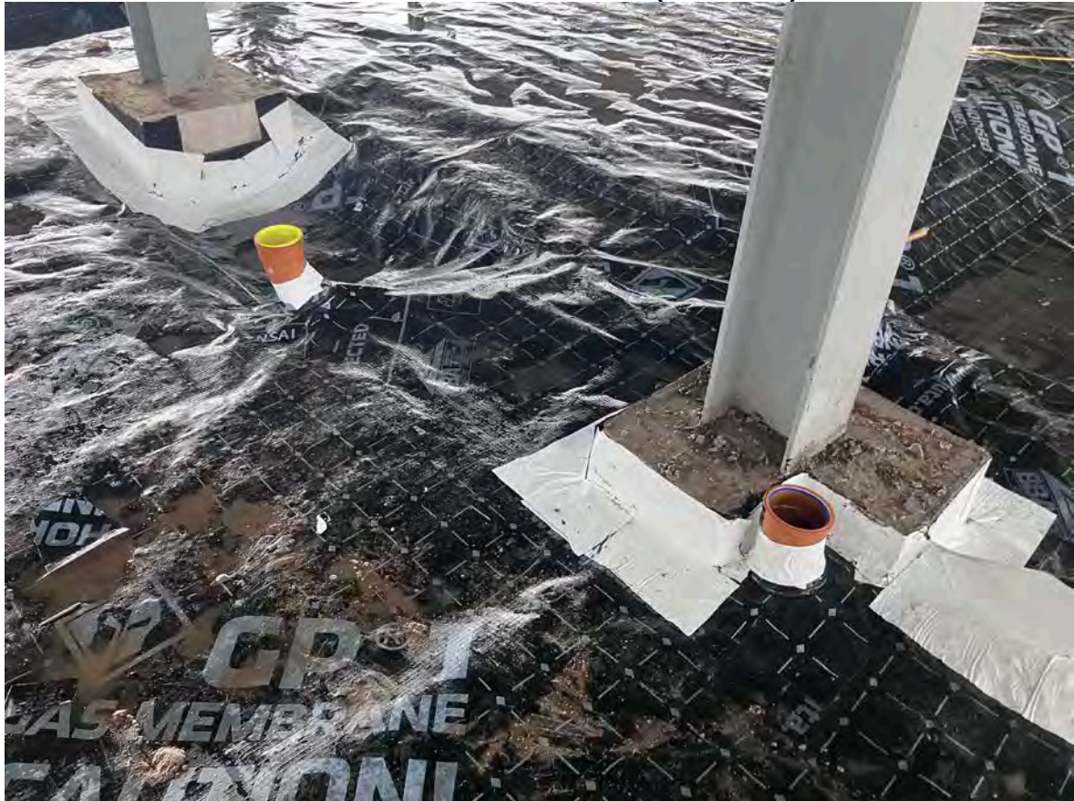
Plate 12 Visit 3 – Area 2 – Edging Detailing and Sealed Penetrations (14/01/25)
