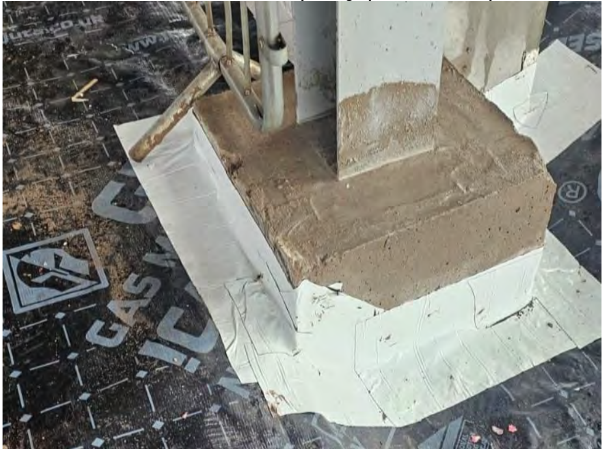
Plate 32 Area 2 – Sealed Penetration (Photograph From Installer)
