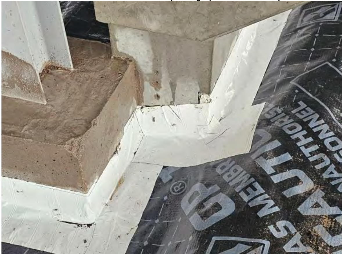
Plate 32 Area 2 – Sealed Penetration (Photograph From Installer)
