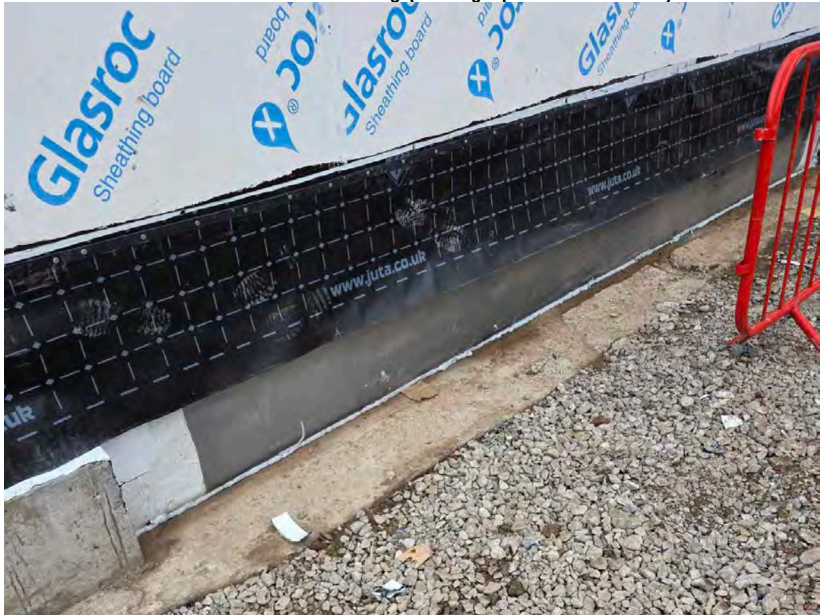
Plate 40 Exterior Perimeter Detailing (Photograph From Installer)
