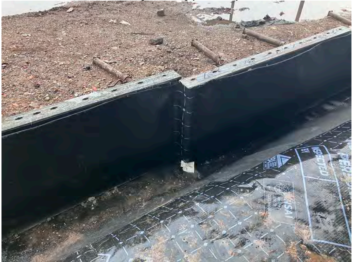
Plate 14 Visit 3 – Area 2 – Membrane Including lift Pit (14/01/25)
