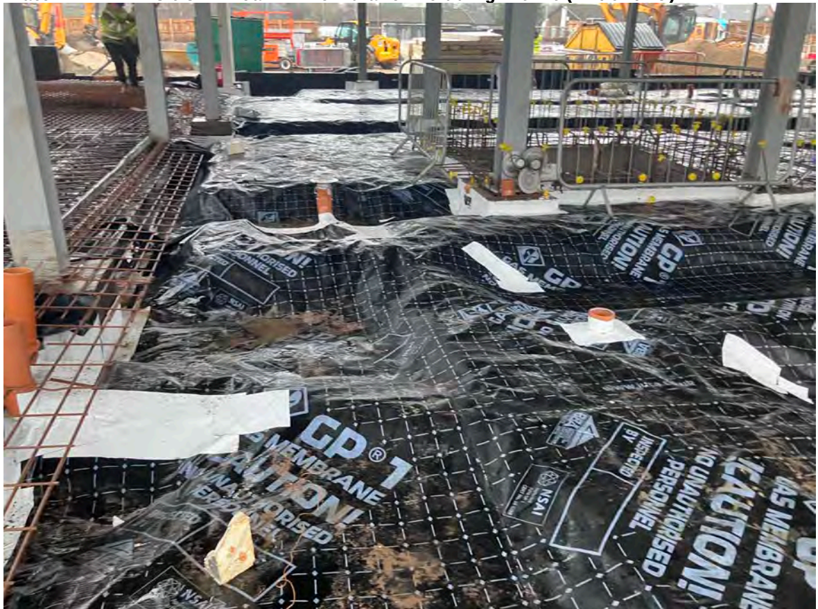
Plate 14 Visit 3 – Area 2 – Membrane Including lift Pit (14/01/25)
