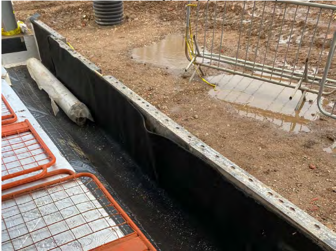
Plate 34 Area 3 – Perimeter and Sealed Penetration (Photograph From Installer)
