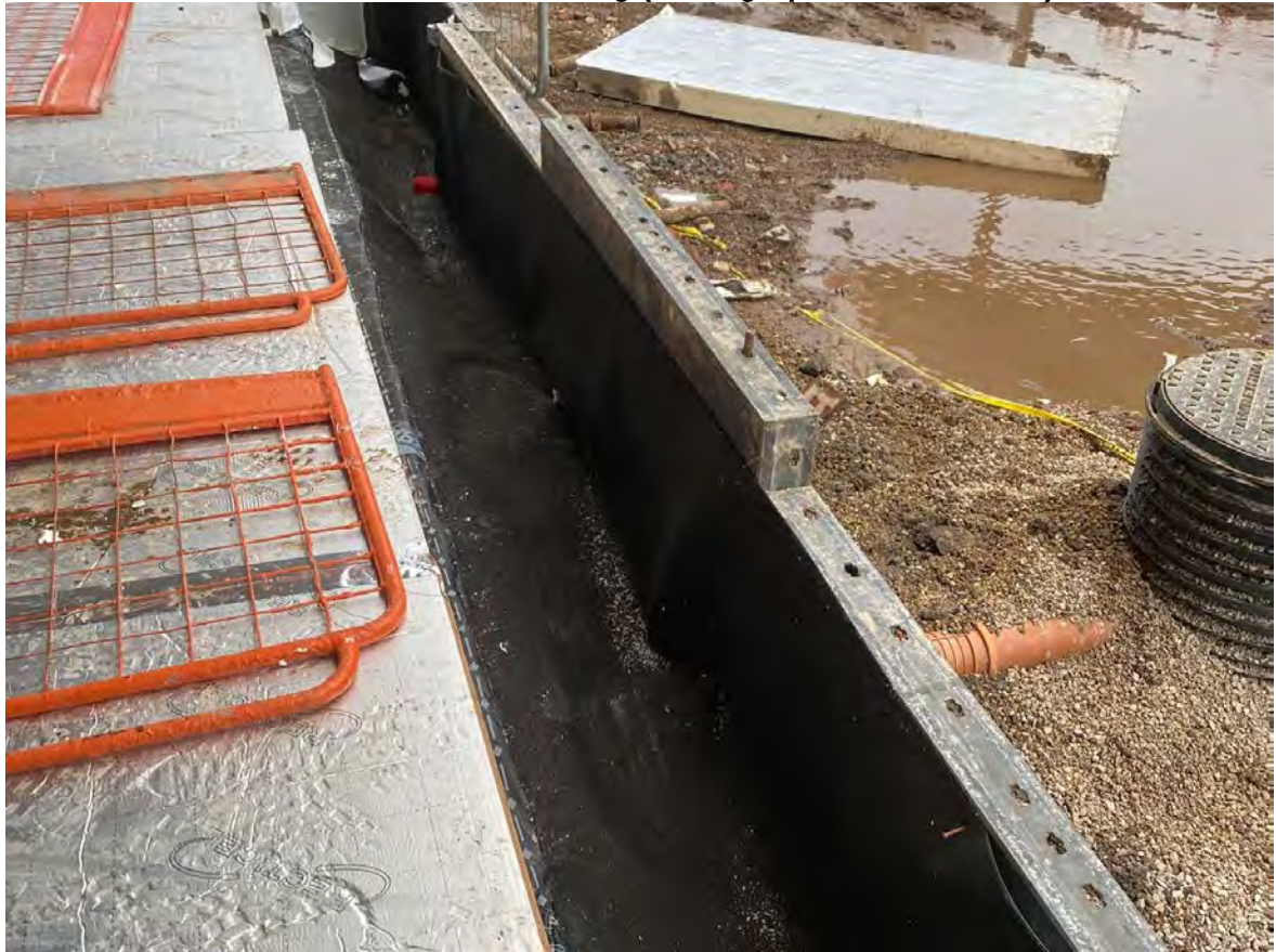
Plate 36 Area 3 – Sealed Penetration (Photograph From Installer)
