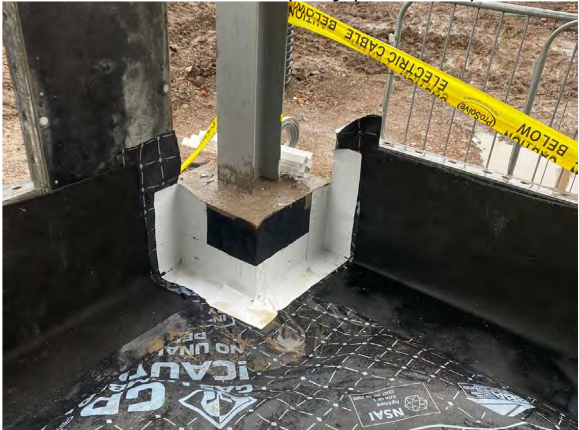
Plate 36 Area 3 – Sealed Penetration (Photograph From Installer)
