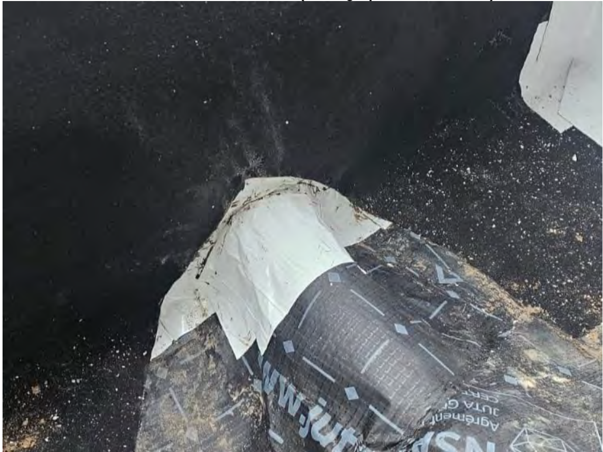
Plate 30 Area 2 – Corner Detailing (Photograph From Installer)
