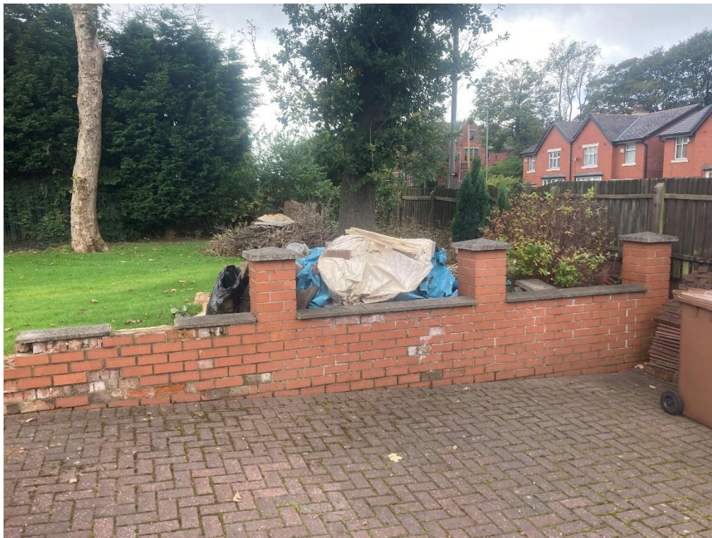
PLATE 3 RETAINING WALL WESTERN CORNER OF SITE
