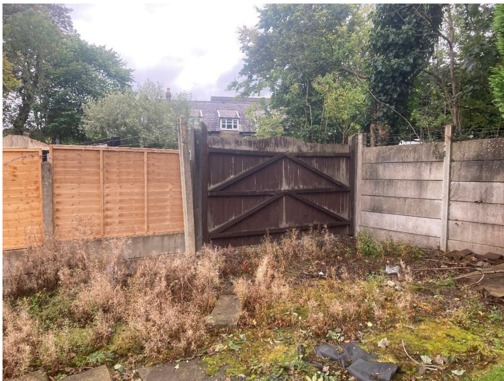
PLATE 4 ENTRANCE TO REAR OF PROPERTY
