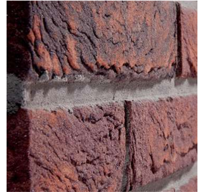
Mortar - Colour matched to each tone (Flush joint to maintain crisp geometry)
