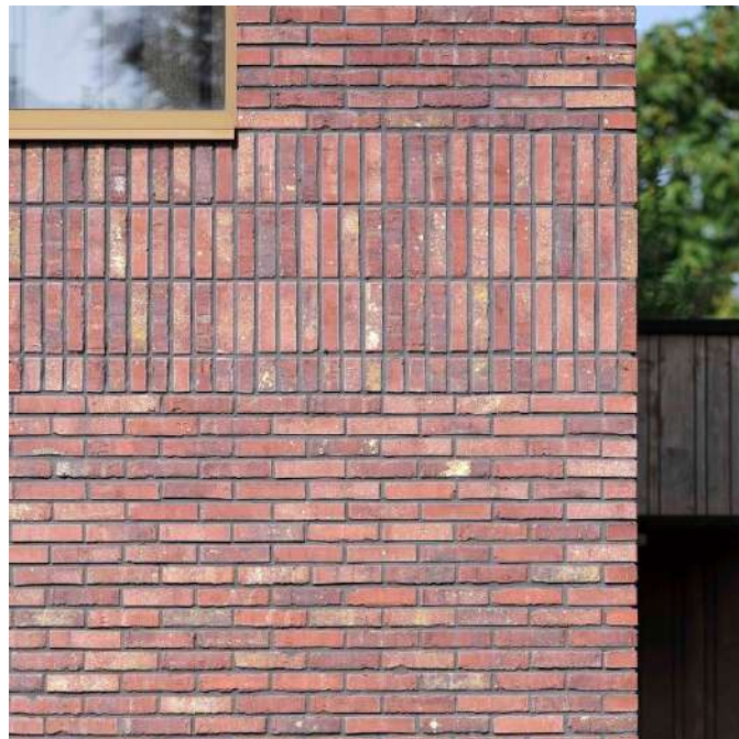
Feature Courses - At first floor break lines
