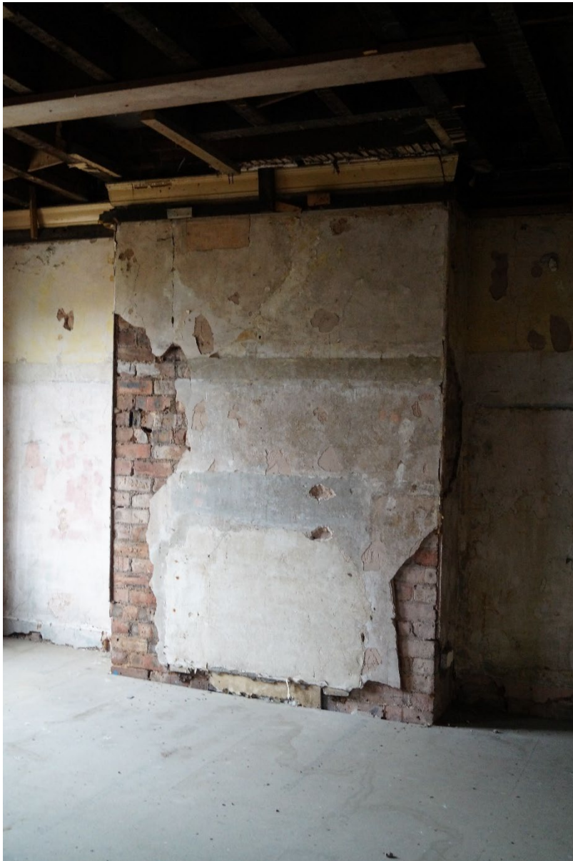
Fig.8: Internal view of the first floor to the rear showing the bare walls and removed ceiling. The projecting bay in the centre of the photograph is a chimney breast and former fireplace position.
