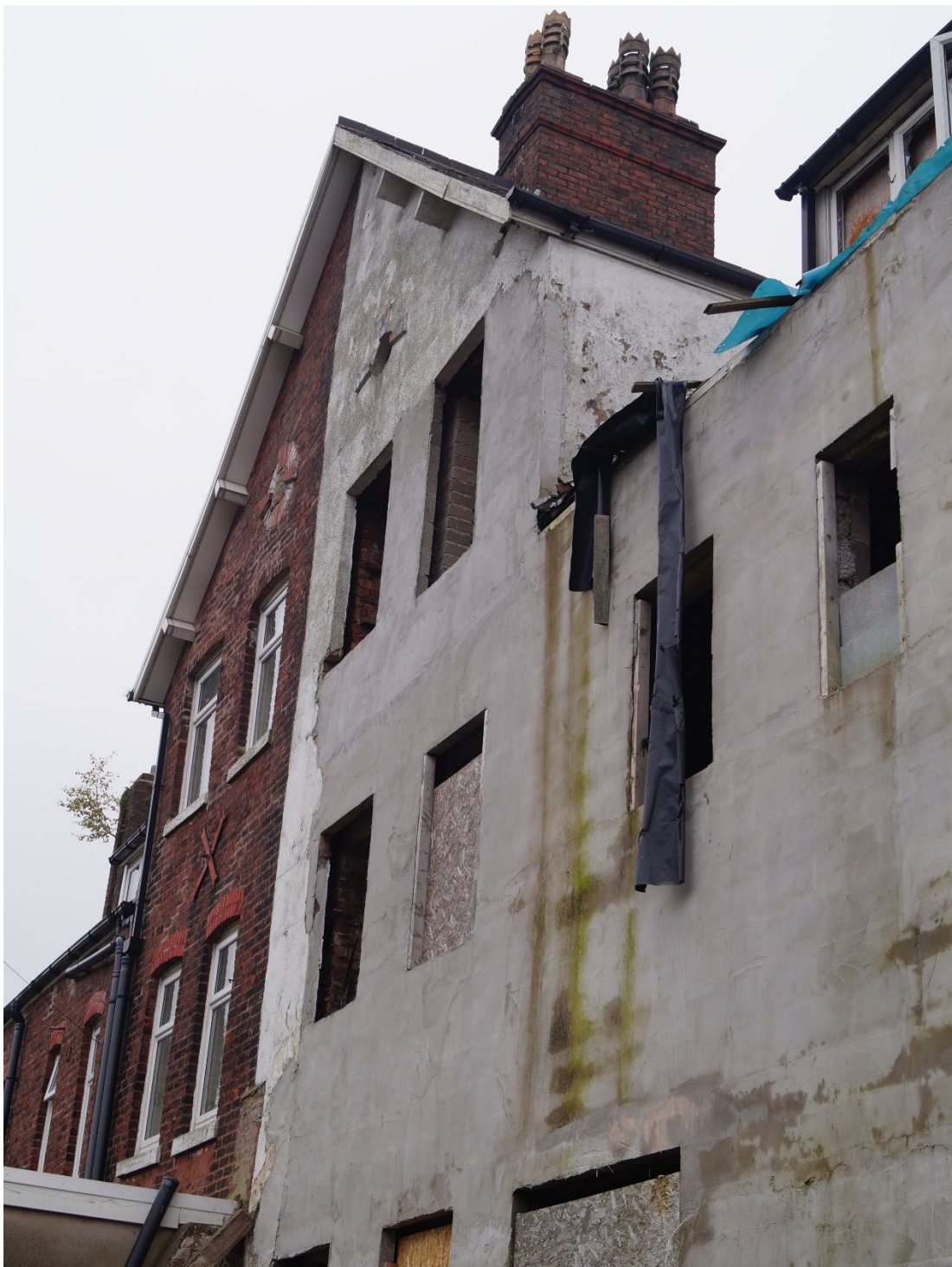
Fig.3: Rear elevation showing the rendered finish and square headed window openings. The adjoining brickwork of 39 Rochdale Road shows the original appearance.
