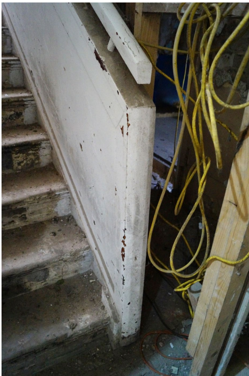
Fig. 9: Internal view of the ground floor at the foot of the stairs. There may be historic context to the balustrading behind the infill panel.
