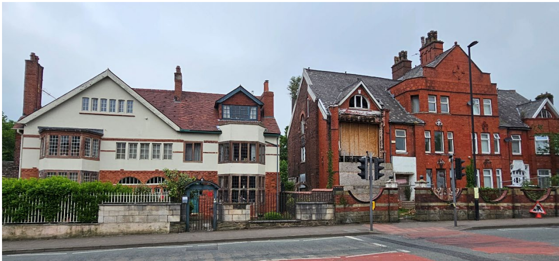
Fig.31: Photograph showing nos.33 and 35 Rochdale Road (left) in context with nos.37 and 39 Rochdale Road (right). The repair of no.37 Rochdale Road would enhance the setting of nos.33 and 35.
