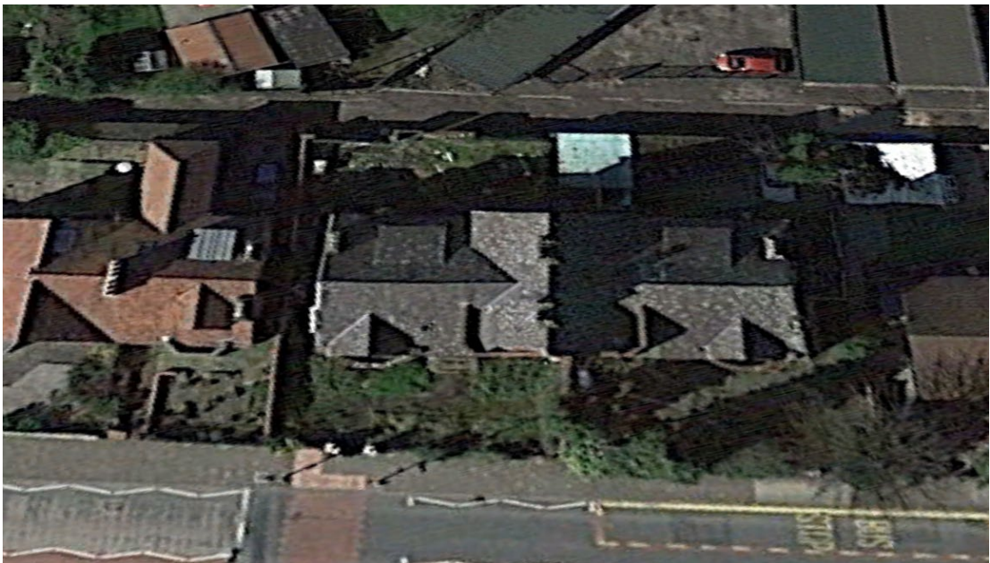
Fig.24: Satellite image of the building from above in 2017 showing the garden overgrown.
