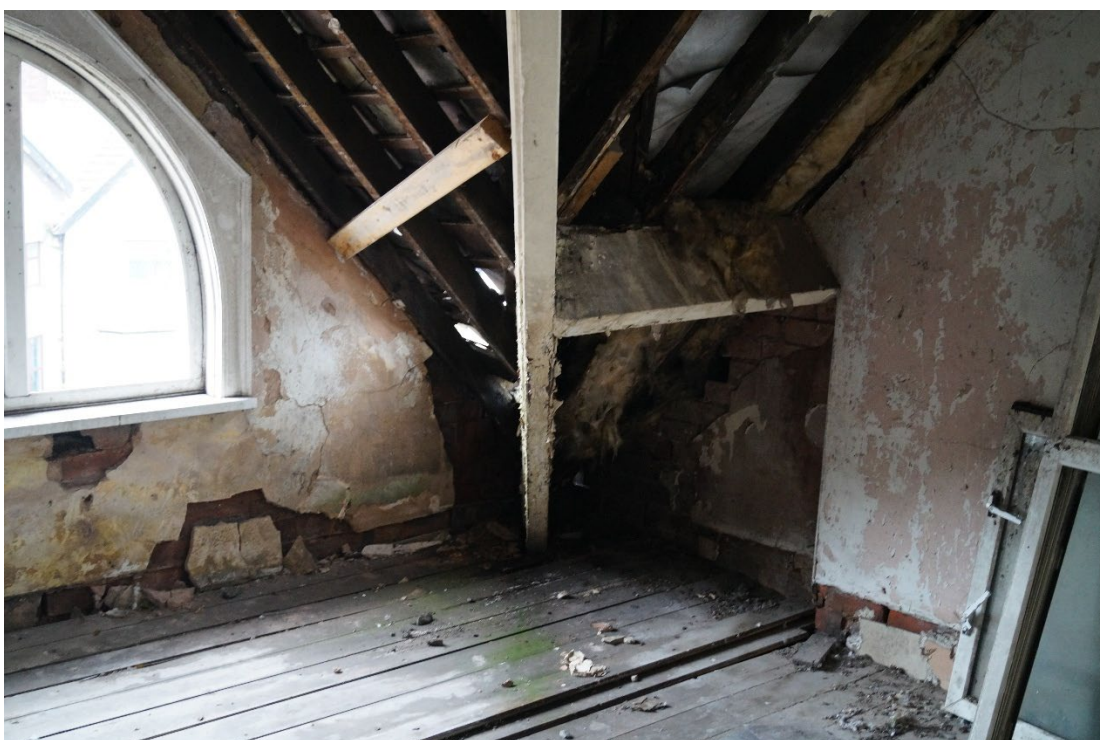
Fig.6: Internal view of the Diocletian window at second floor level showing daylight visible to the valley.
