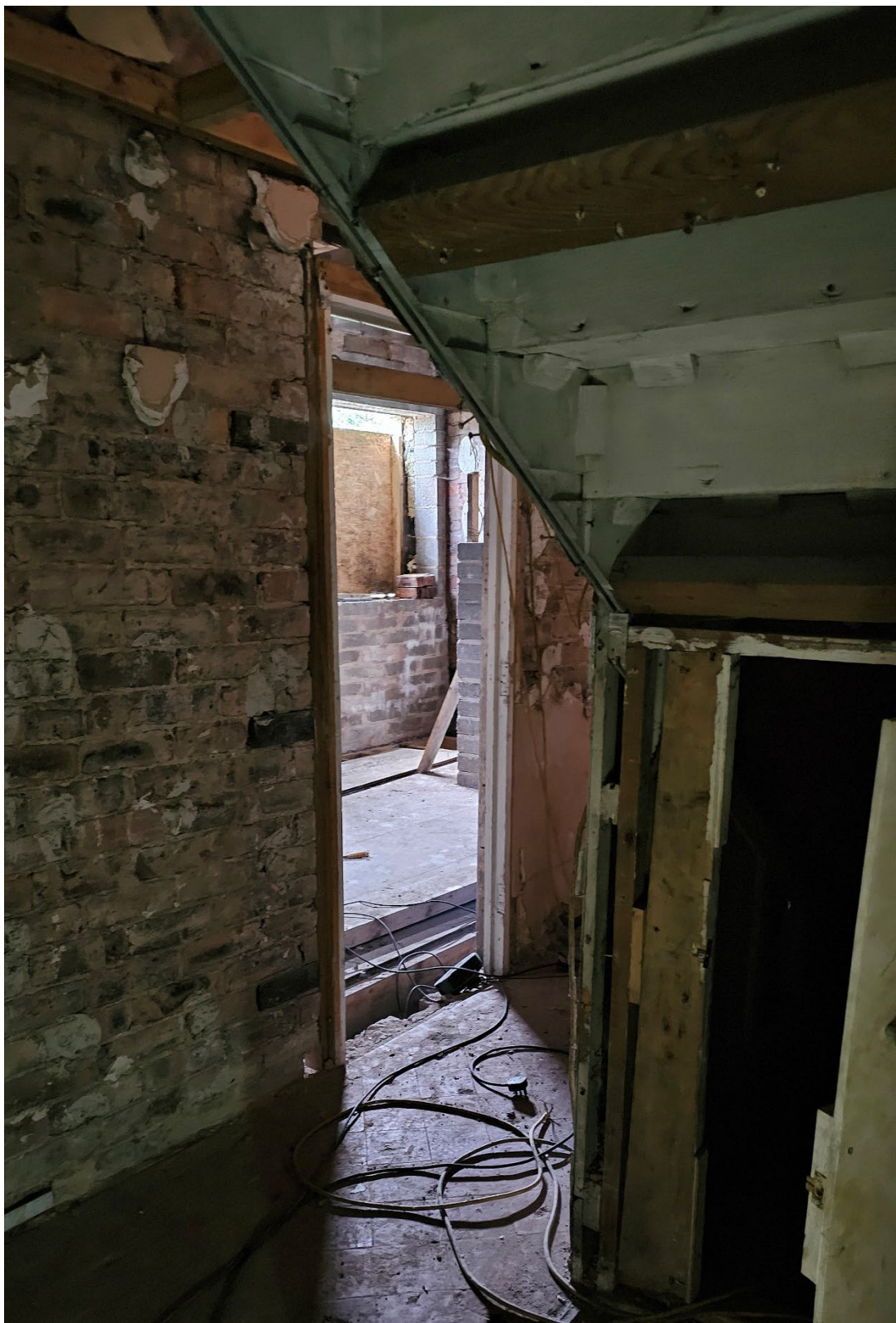
Fig.12: Internal view of ground floor beneath the stairs looking towards the rebuilt rear wall.
