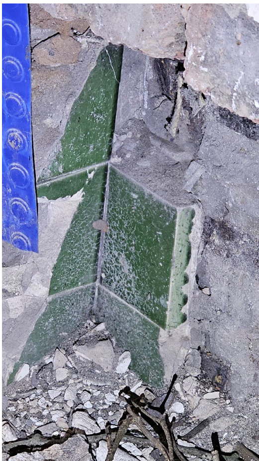
Fig. 10: Internal view of the fragment of green hearth tiles remaining to ground floor front room, which will be replicated as closely as possible in new tiles for reinstating the fireplace in this room.
