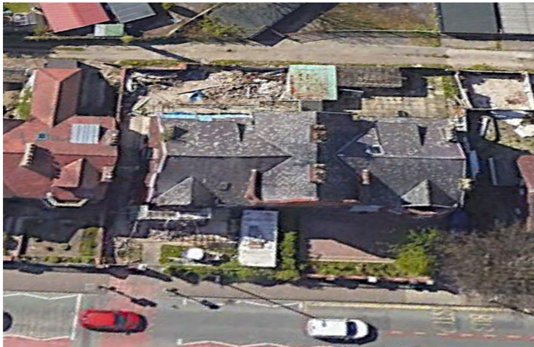
Fig.26: Scaffolding present in this satellite photograph of April 2022, indicating the dismantling of the bow window. The flat roof structure to the front garden is presumed to be the site office for the contractors.
