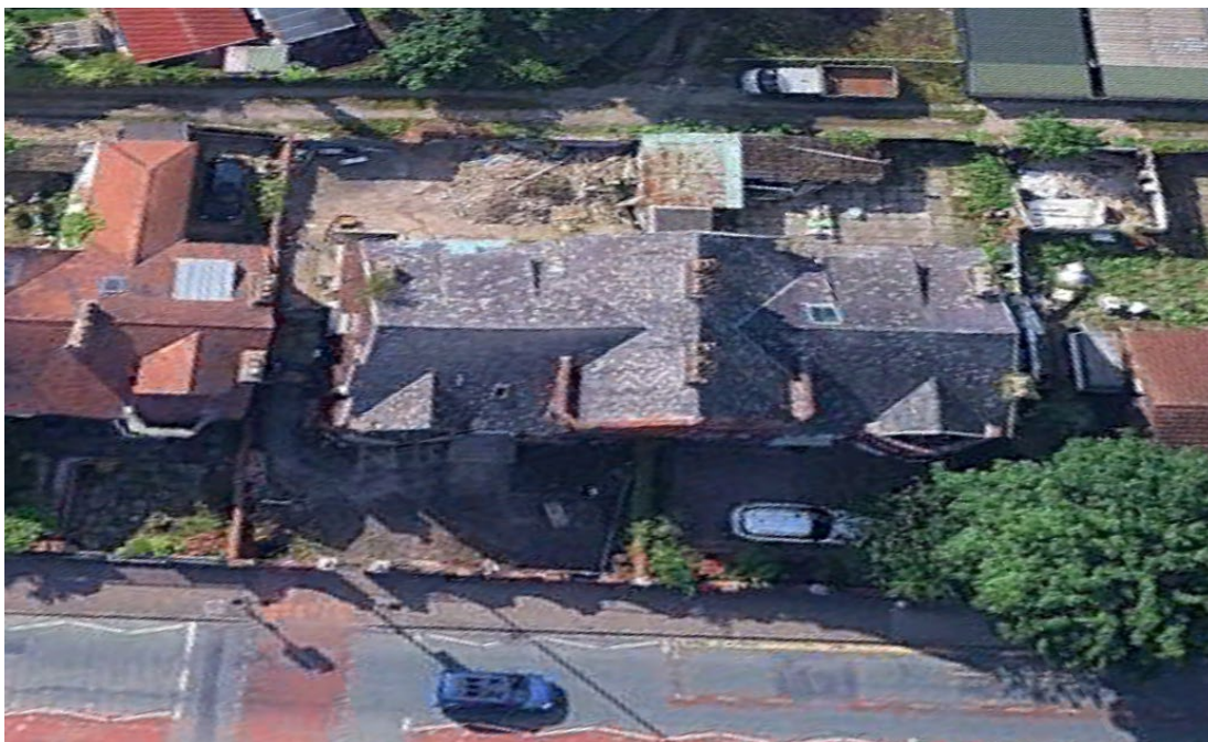
Fig.27: The windows to the bow are no longer visible in this satellite photograph of June 2023, indicating the bow window is no longer in situ.
