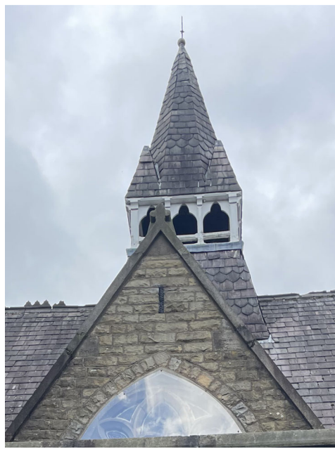
Cupola, East side Cupola wooden undamaged; requires further inspection
