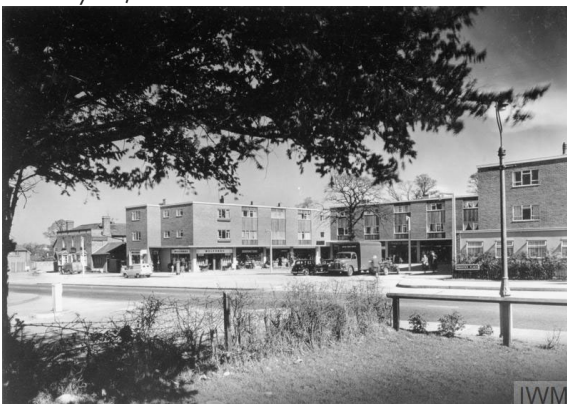
Figure 3.25 Photograph of the Harlow New Town (Source: www.iwm.org.uk , accessed 11 th February 21)
