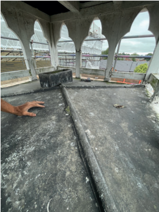
Lead roof looks to be on good condition and does not require renewal. All wraps to timber ends should be in lead.
