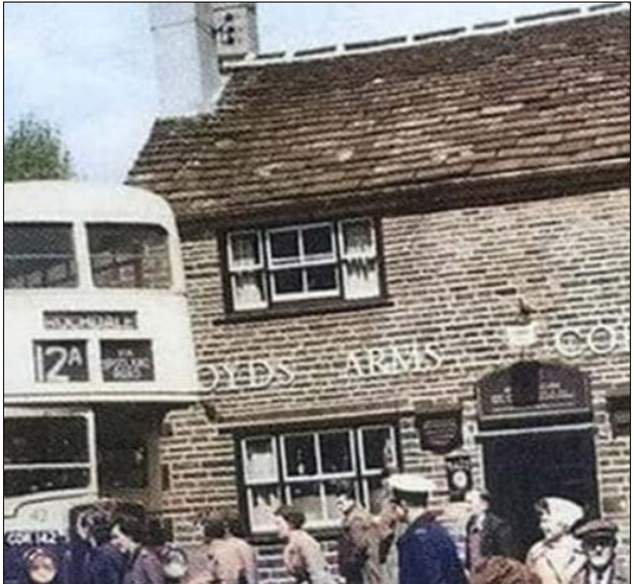
4. Probably 1960s image showing the building prior to alteration in the late 20 th century
