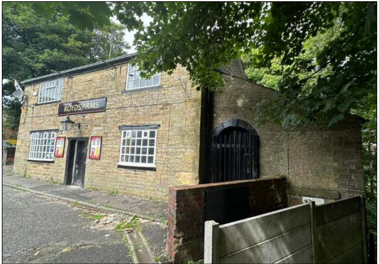
5. The building has now lost its original windows along with its chimneys
