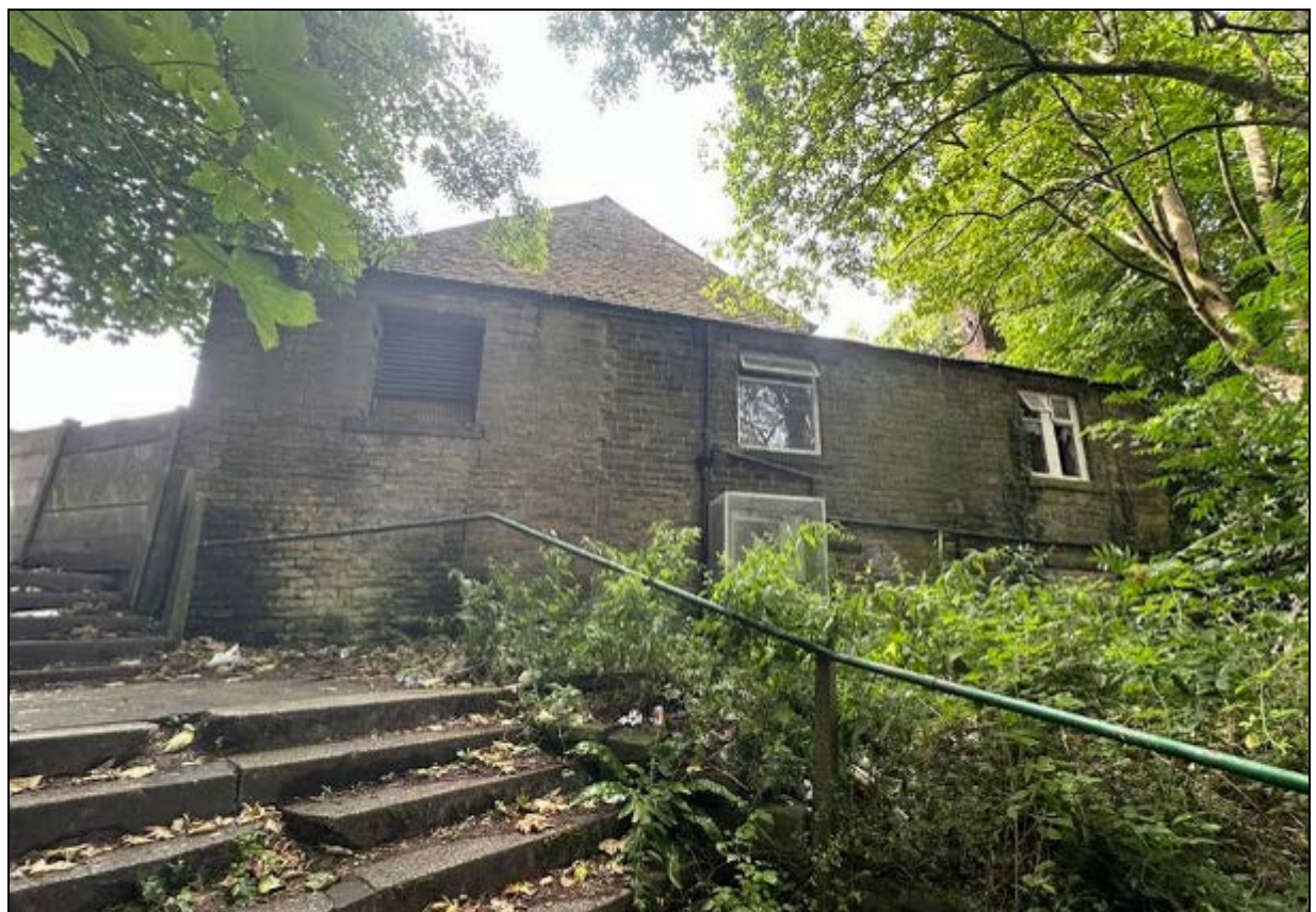
6. View from the east, showing 19 th century side and rear extensions built in two phases
