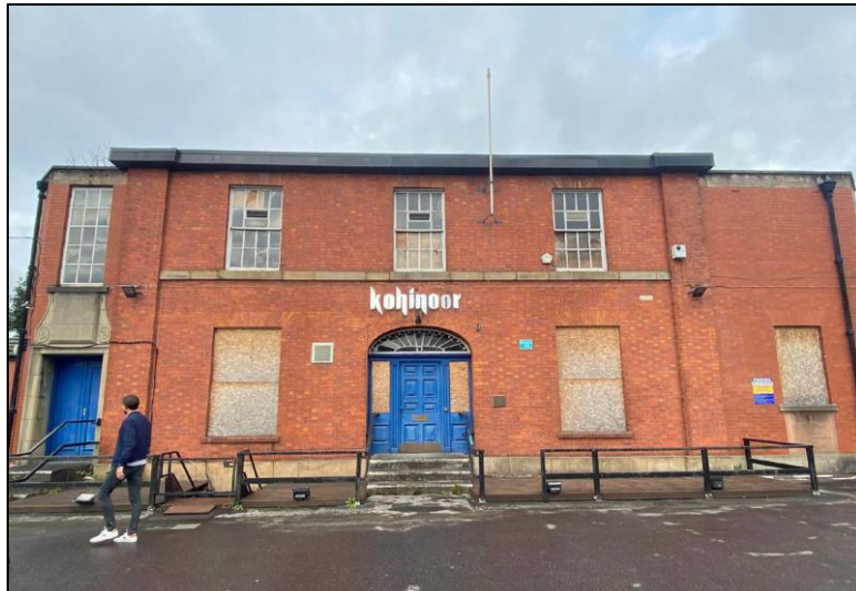
Figure 2 - Frontage of the existing building.
