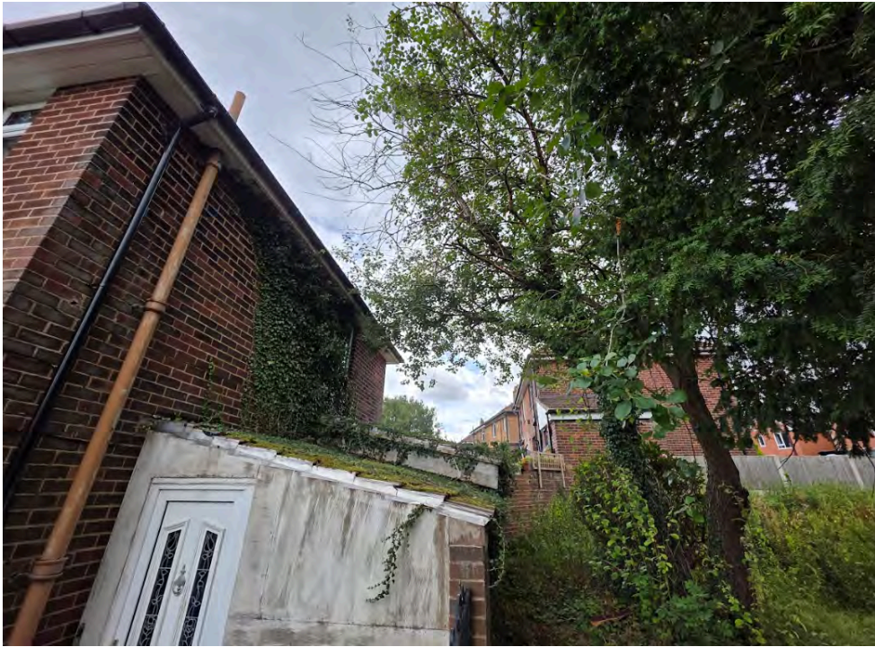
Photographic plate showing the proximity of the existing side extension to T1 & T2 . (ROAVR, 2025)
