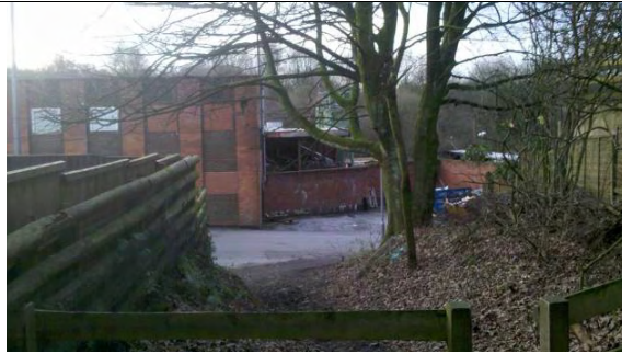
View south from southern end of footpath which bounds west of site. Trows house (off site) to east. Die cast works with bulk storage tanks opposite on south of Trows Lane
