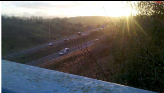
A627 (M) viewed from footbridge at end of Cripple gate Lane near northeast corner of site.
