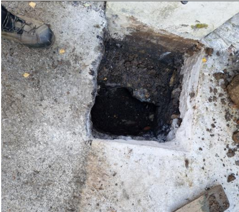
Excavated Hole adjacent to gate post at formation level
