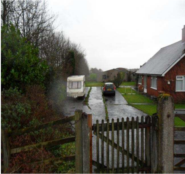
Photo 5: Ginnell Farm buildings in south-eastern part of the site.
