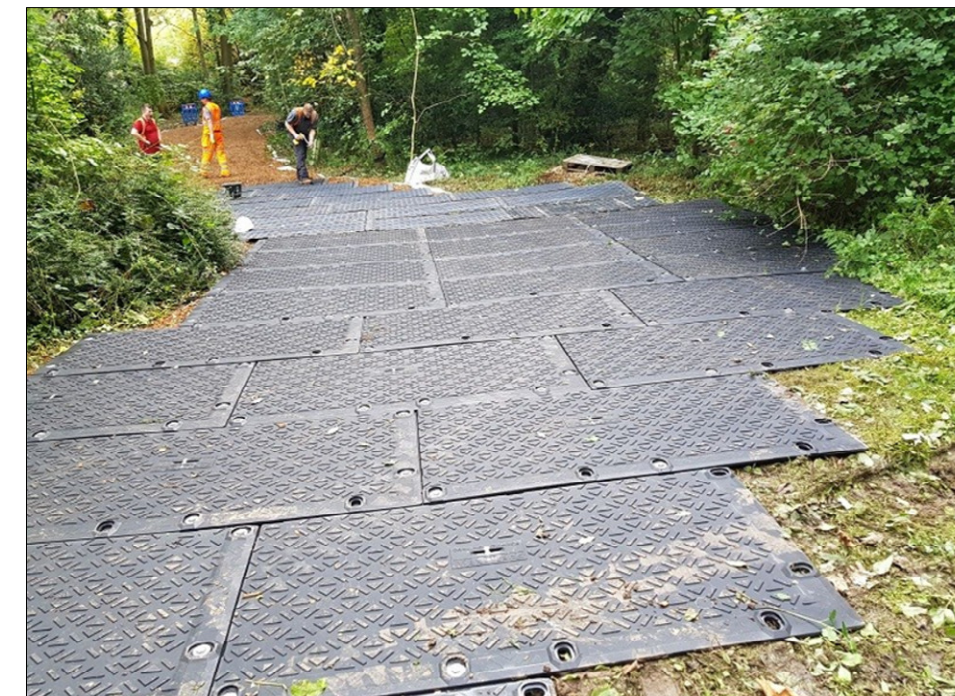
Ground protection boards
