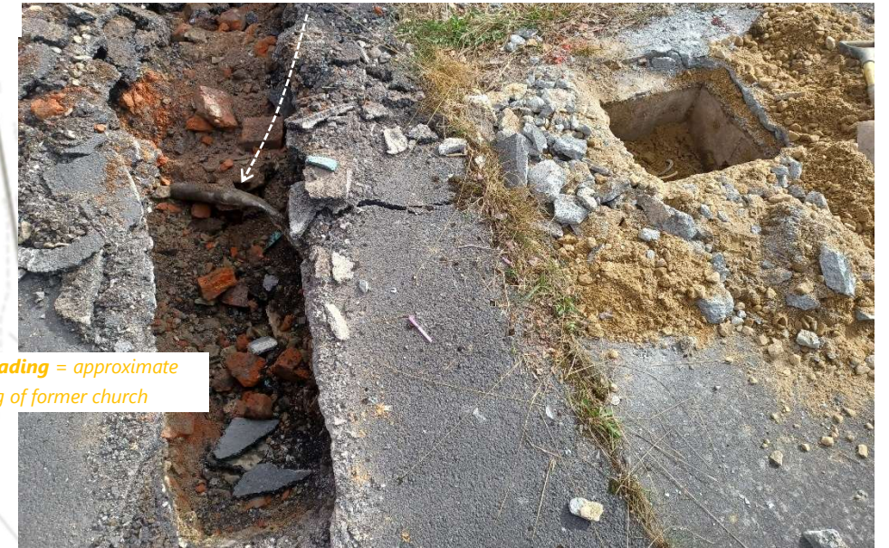
^^ Photograph 3: TP105 and utility box in Photograph 1 – facing eastwards
