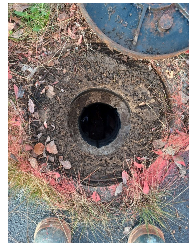
^^ Photograph 4: Drain cover with inspection chamber (?) – invert = 0.65 mbgl. No evidence of fuel odours or staining
