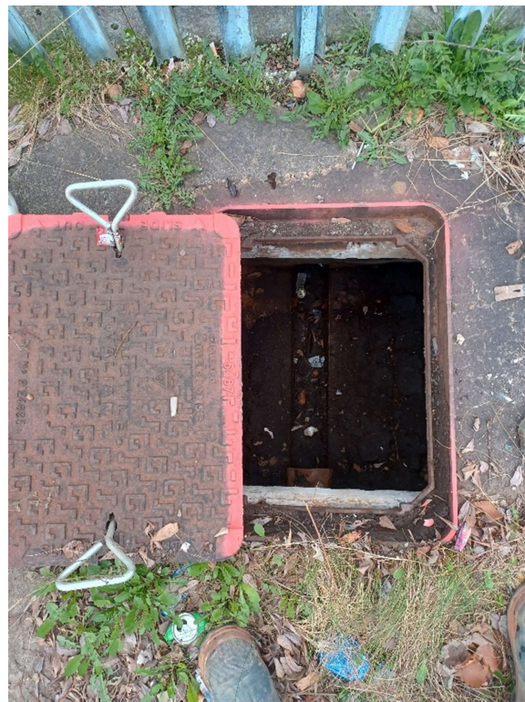
^^ Photograph 2: Drain cover with pipe flow towards Oldham Road – invert = 0.97 mbgl. No evidence of fuel odours or staining
