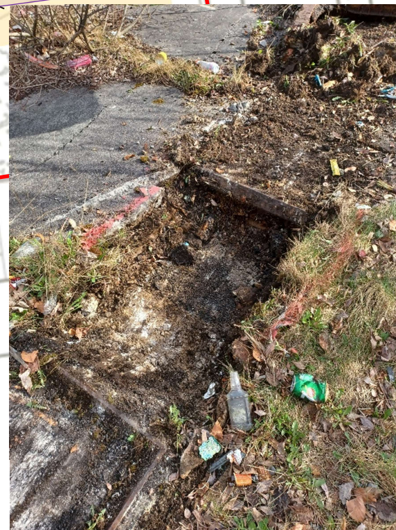
>> Photograph 5: Infilled access cover chamber. No evidence of fuel odours or staining.
