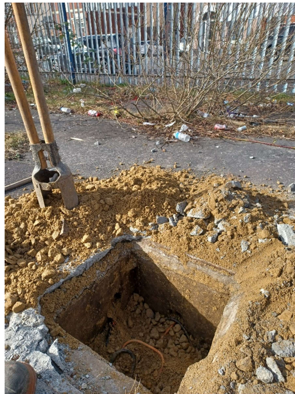
^^ Photograph 1: Utility box likely serving as power to the fuel pumps – no trace on CAT4+
