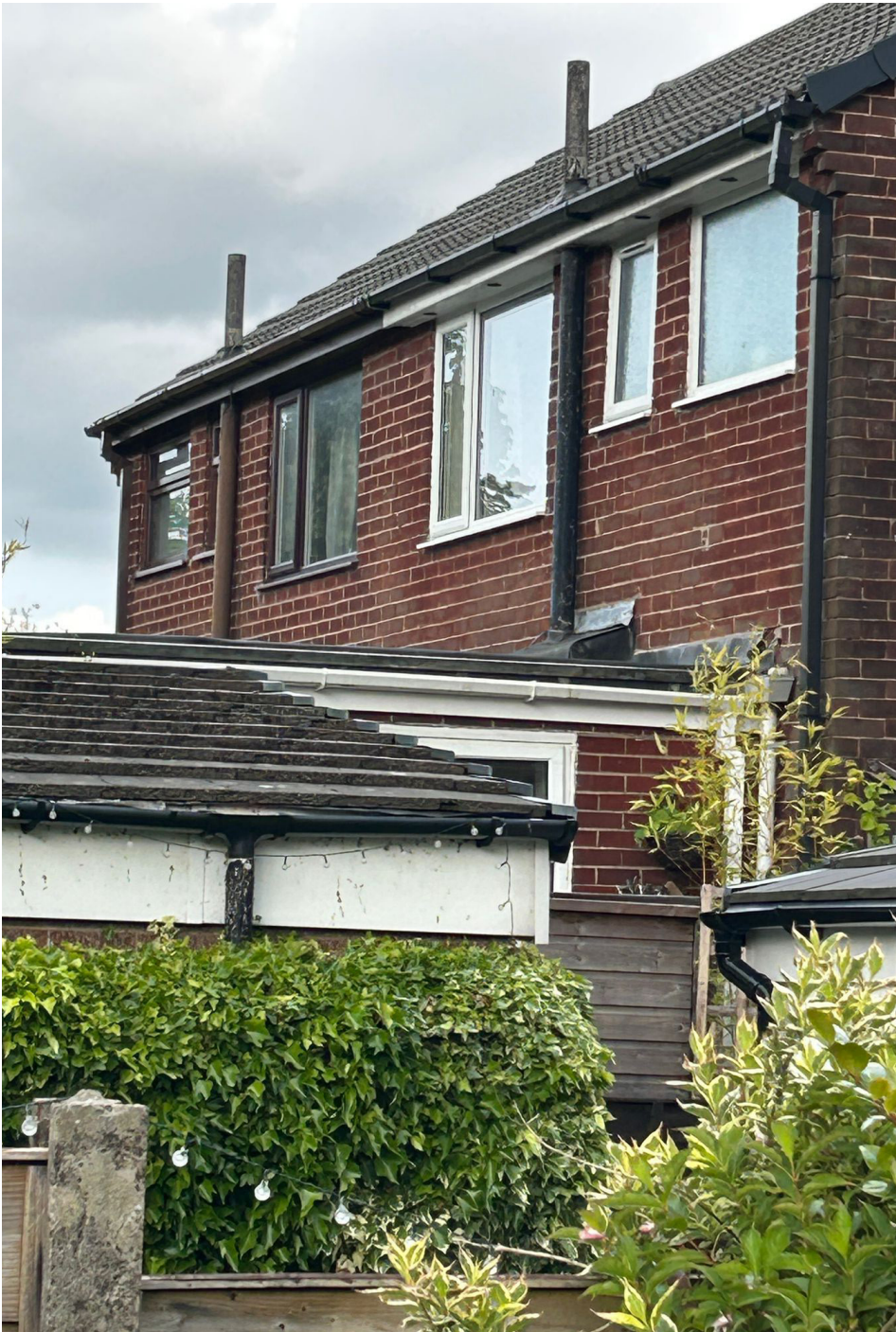
Fig 9. Flat roof rear extension at no.28
