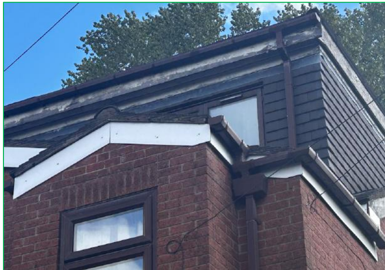
Showing the roof structure of the building adjacent to the north, with well-fitted hanging tiles and fascias.
