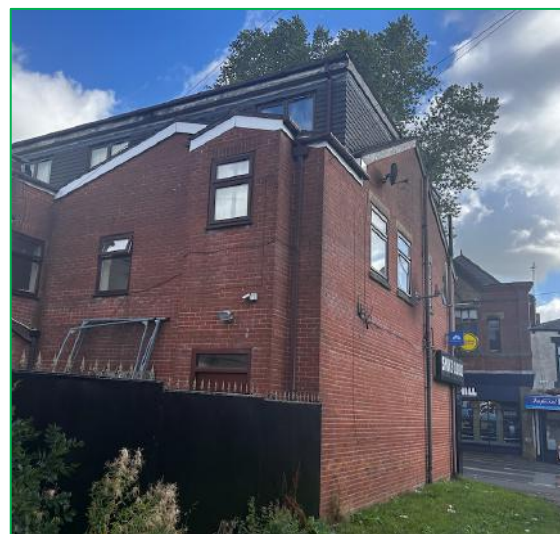
The building to the north
