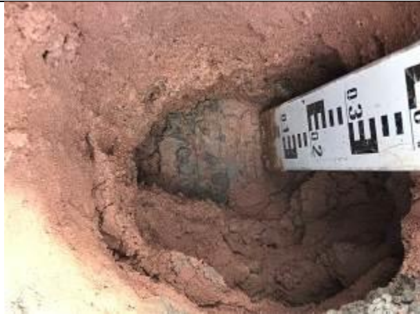
View of soil in capping layer excavation.
