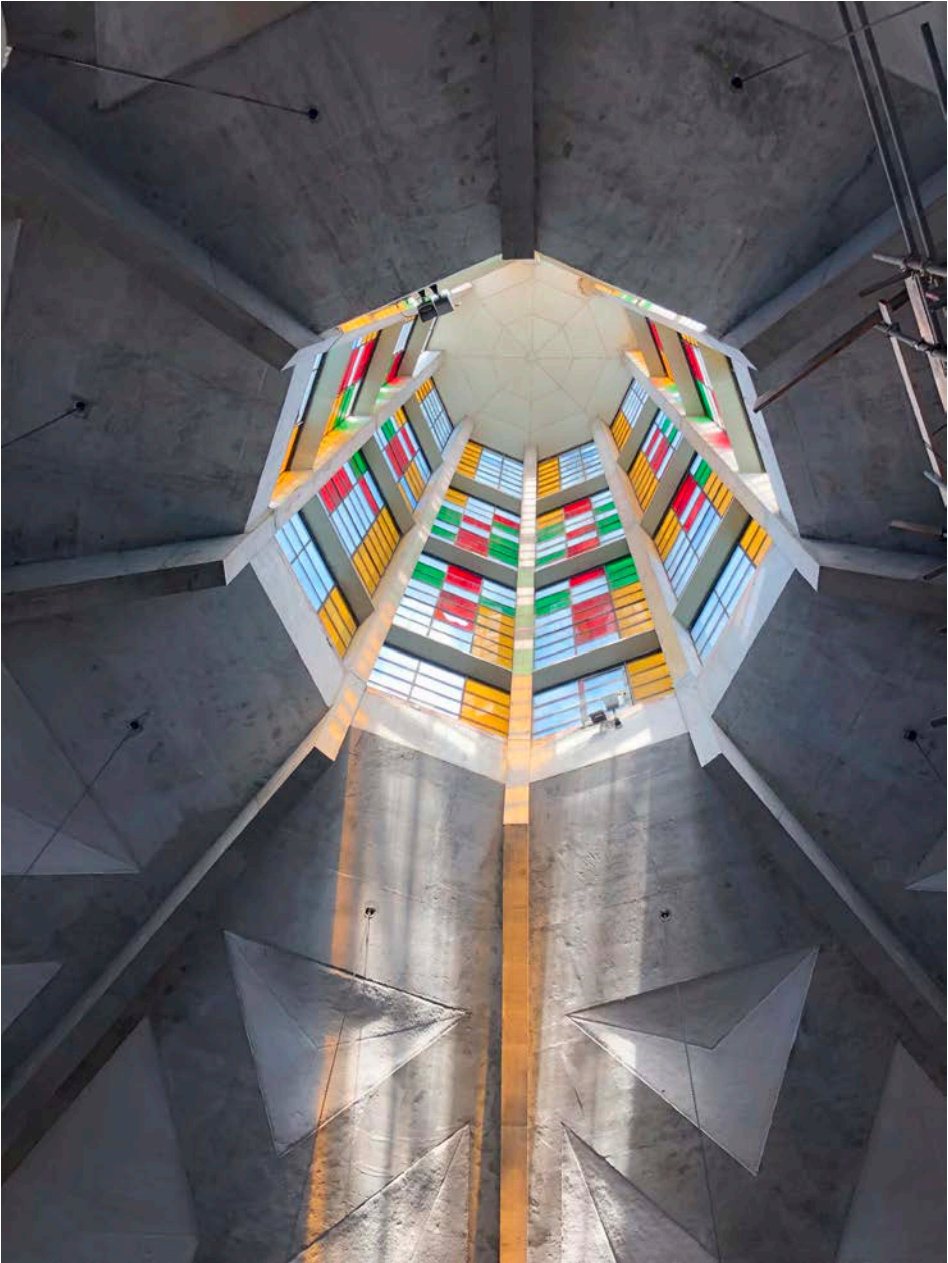
129 View towards Glazed Lantern
