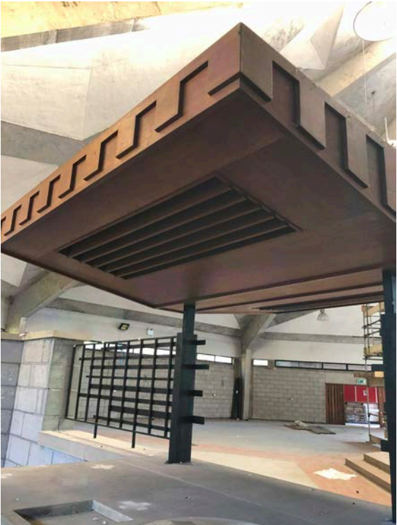
135 View of Ciborium to Blessed Sacrament Chapel
