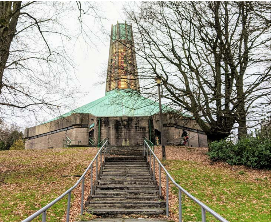
4 View from the existing stepped access up the hill towards the building from the East
