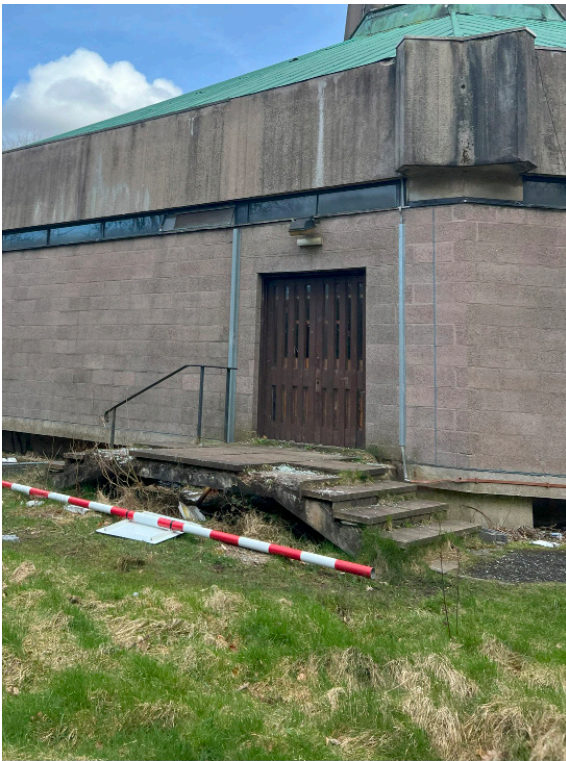
48 View of Steps to West Porch
