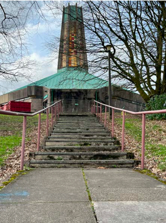
43 View of External Steps to East
