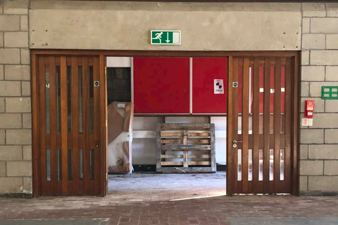
155 Internal Doors between Narthex and Chapel
