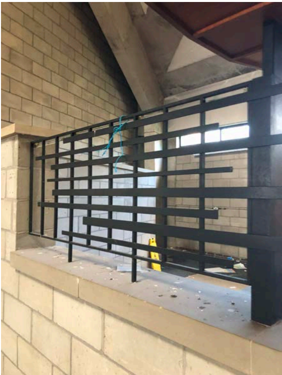
138 View of Metal Screen to Blessed Sacrament Chapel
