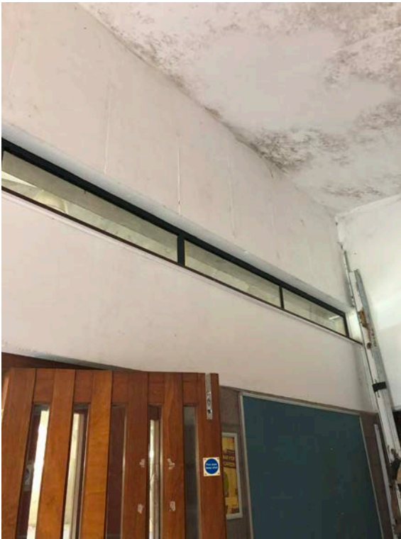
161 Internal Clerestory Windows viewed from within Narthex
