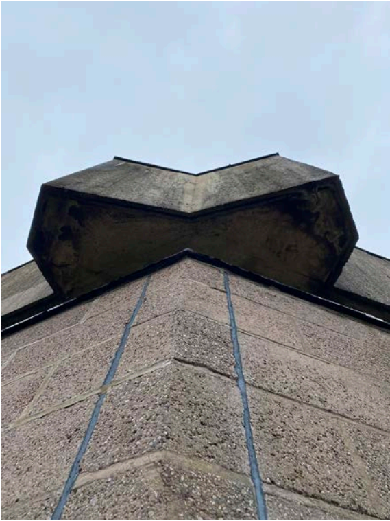
21 Detail of Concrete Structure
