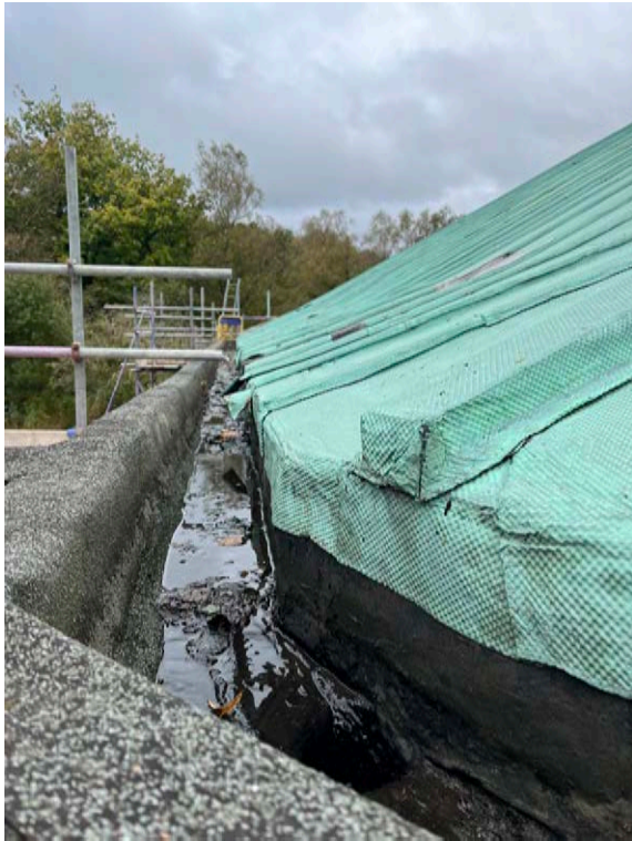
32 Parapet Gutter Detail
