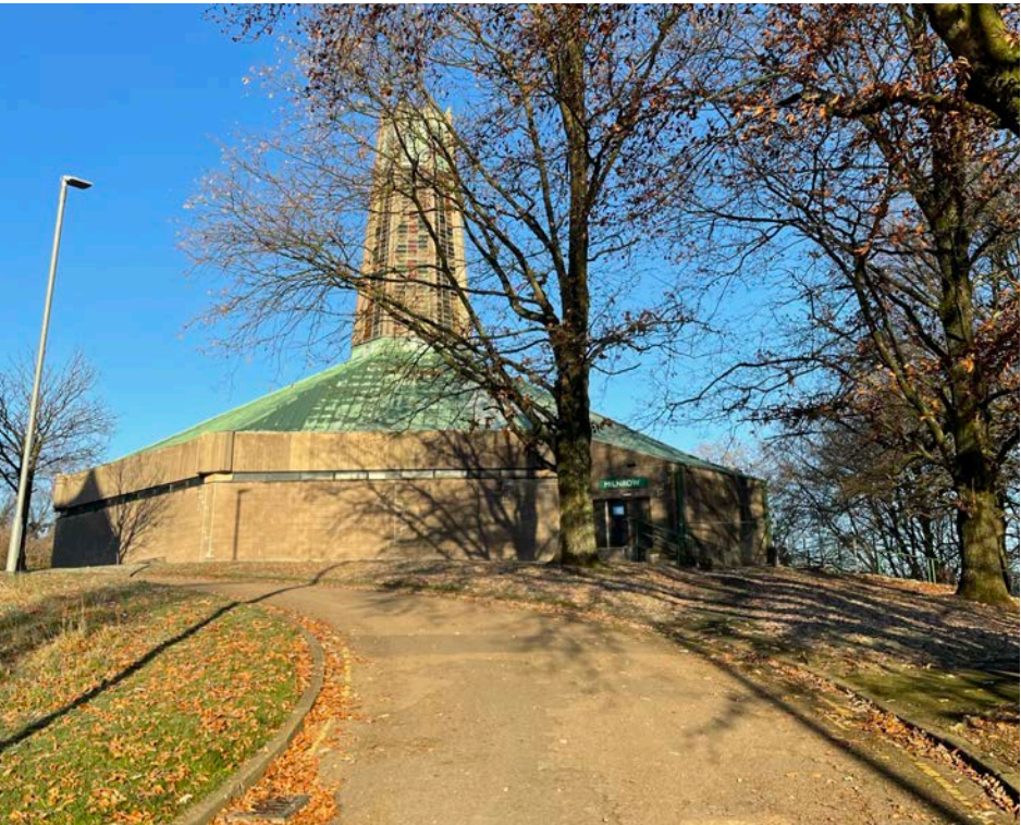
5 View from the existing stepped access up the hill towards the building from the South-East
