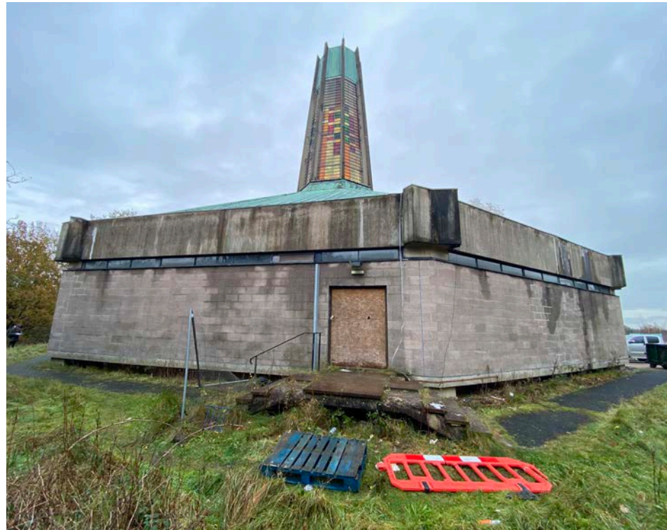
6 West Elevation Looking Towards the West Porch
