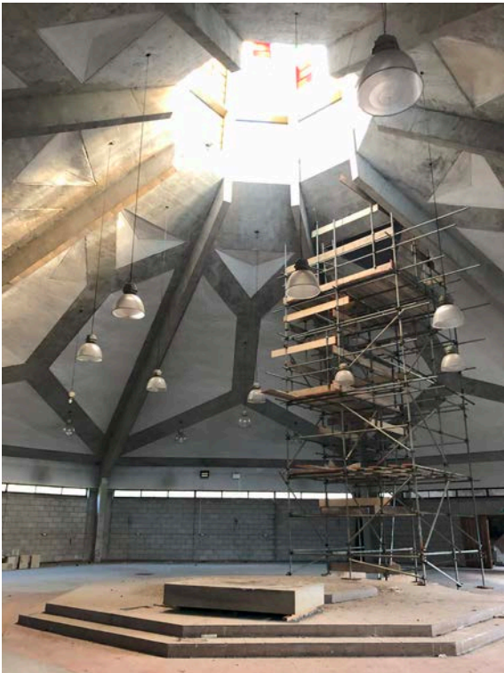
131 View towards Sanctuary showing relationship between Sanctuary and glazed lantern
