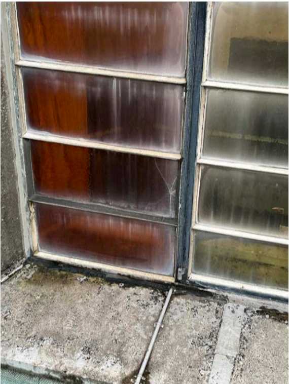
42 Detail of Glazed Lantern
