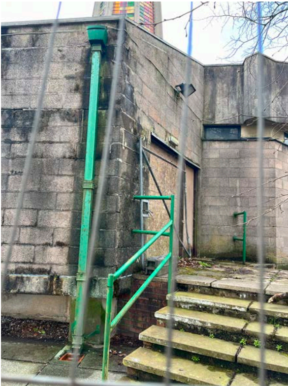
17 View from the existing stepped access up the hill towards the building from the South-West
