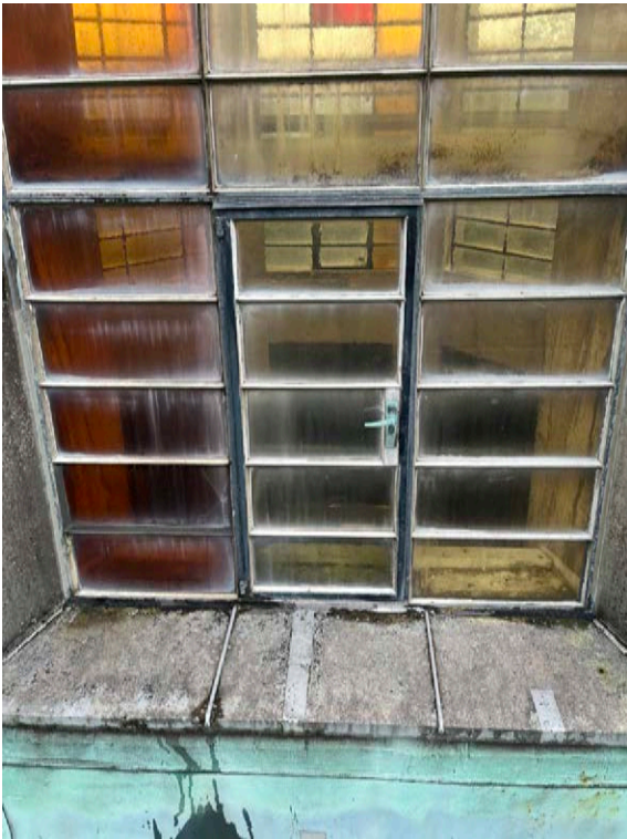
40 Detail of Glazed Lantern
