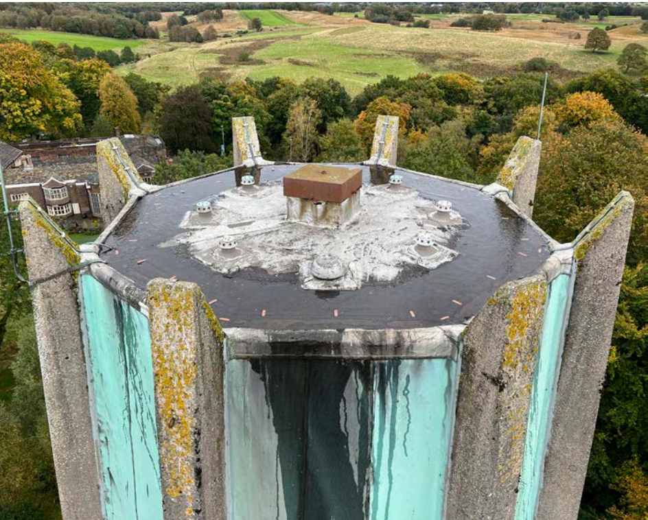
39 View of flat roof to top of Lantern
