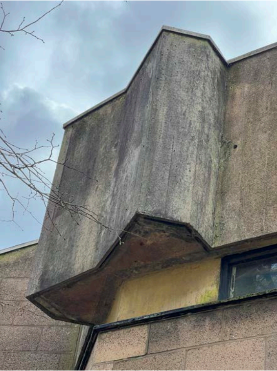
20 Detail of Concrete Structure
