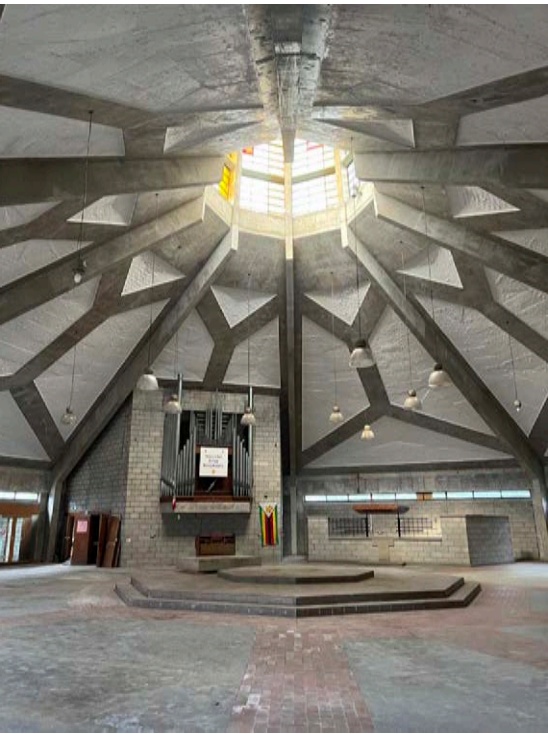
186 View towards Sanctuary and Pipe Organ
