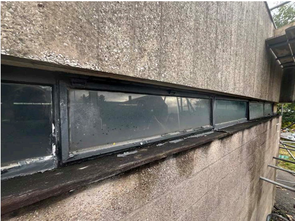
27 View of Clerestory Windows
