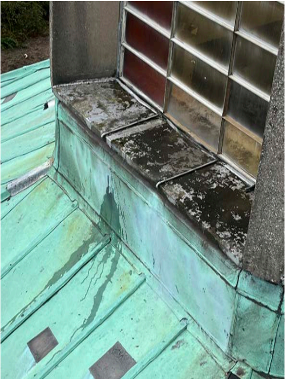
38 View of Base of Glazed Lantern
