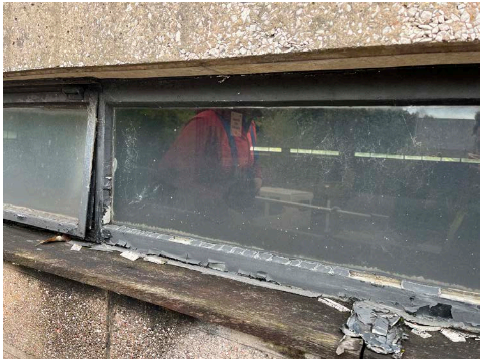
29 View of Clerestory Windows
