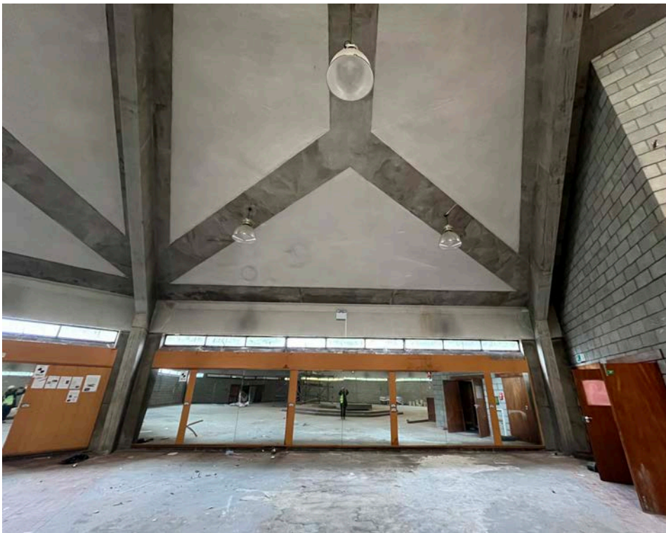
113 View of Chapel with later addition wall covering
