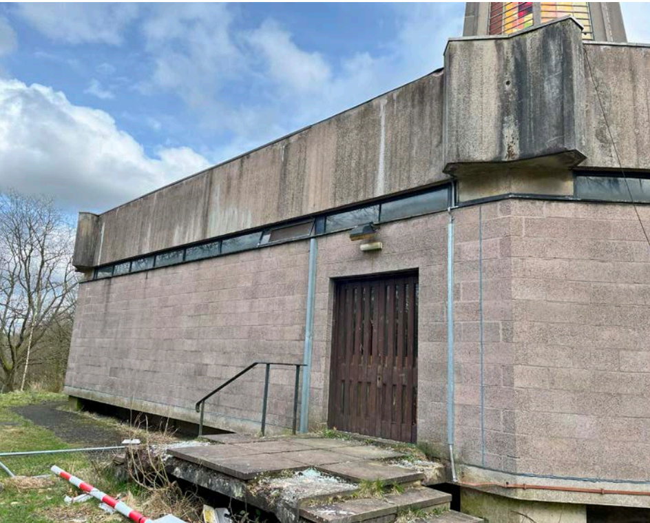
10 West Elevation looking towards the West Porch
