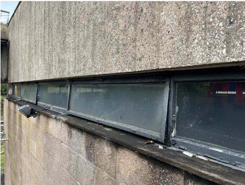
28 View of Clerestory Windows
