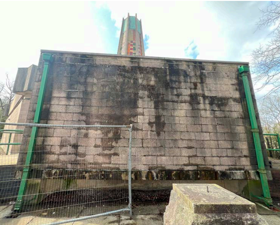
16 View from the existing stepped access up the hill towards the building from the South-West
