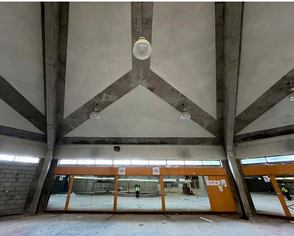
112 View of Chapel with later addition wall covering
