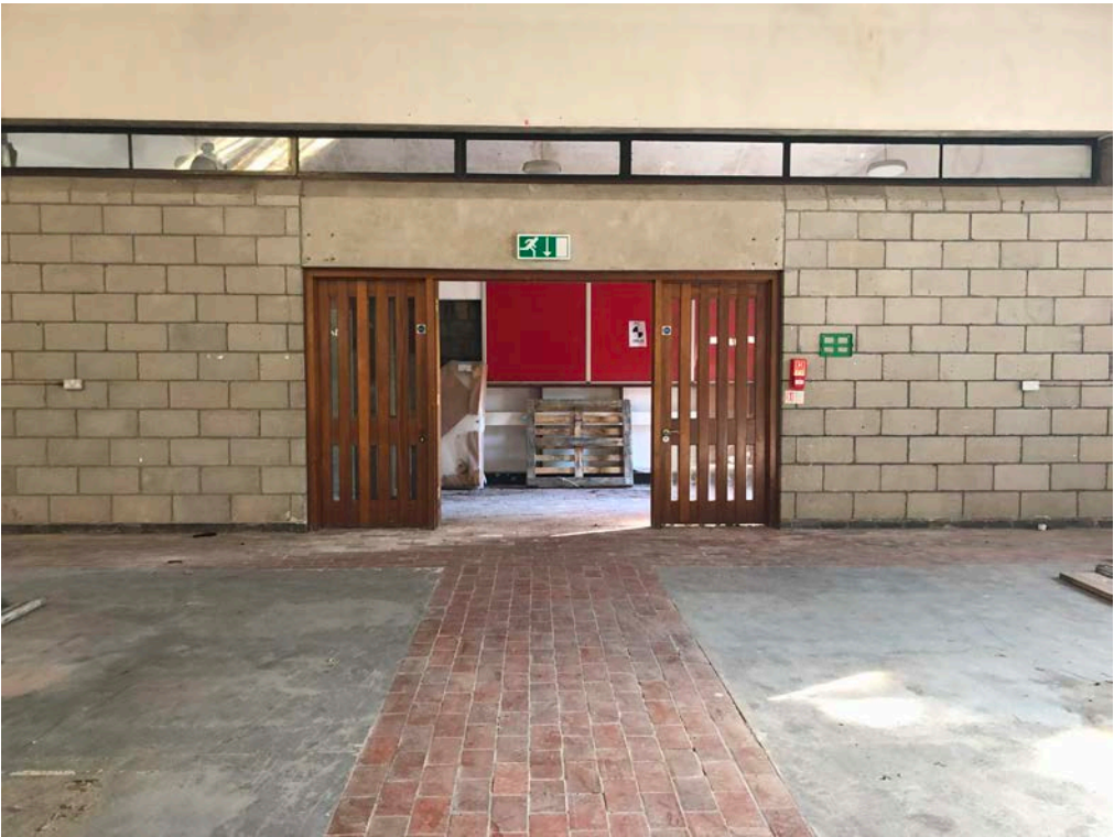
160 Internal Clerestory Windows viewed from within Chapel
