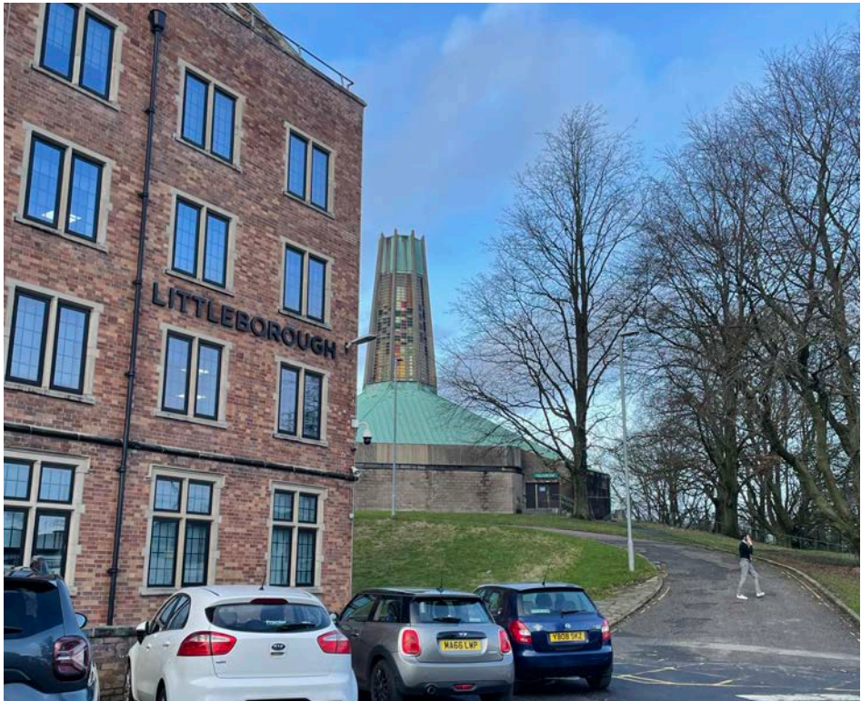
3 View towards the Chapel from within the Hopwood Hall College campus
