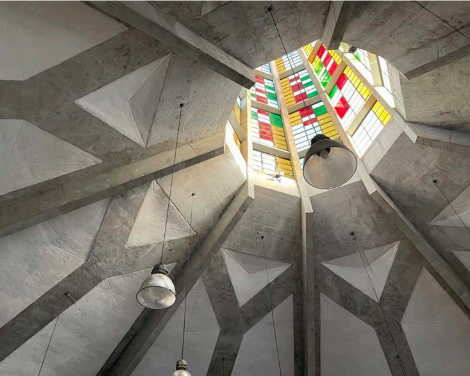
127 View towards Glazed Lantern
