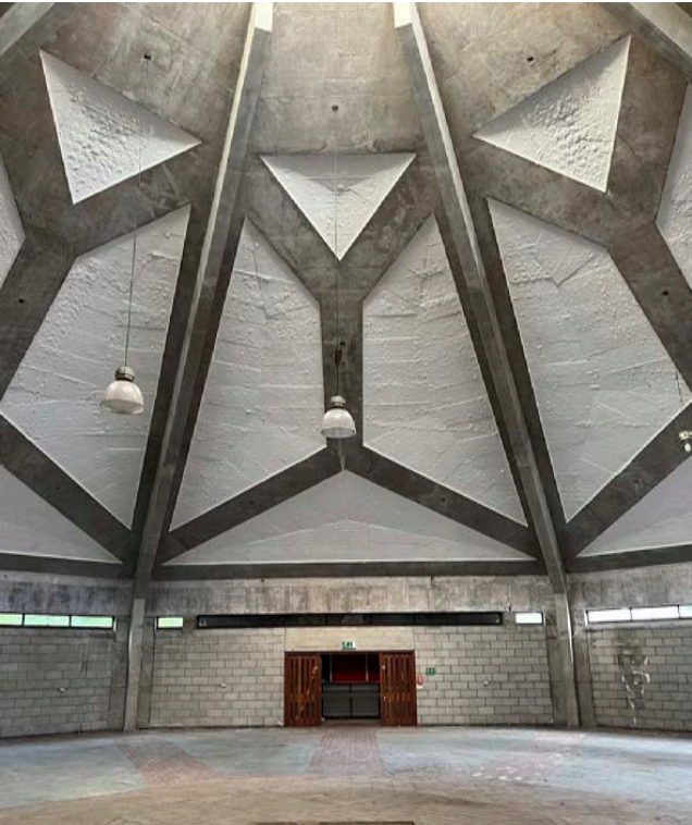
174 View Towards Sanctuary and Main Entrance Doors into Chapel
