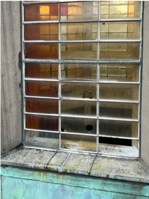
41 Detail of Glazed Lantern
