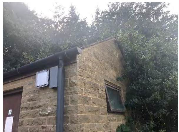
Figure 22. Sealed gable of the existing toilet block
