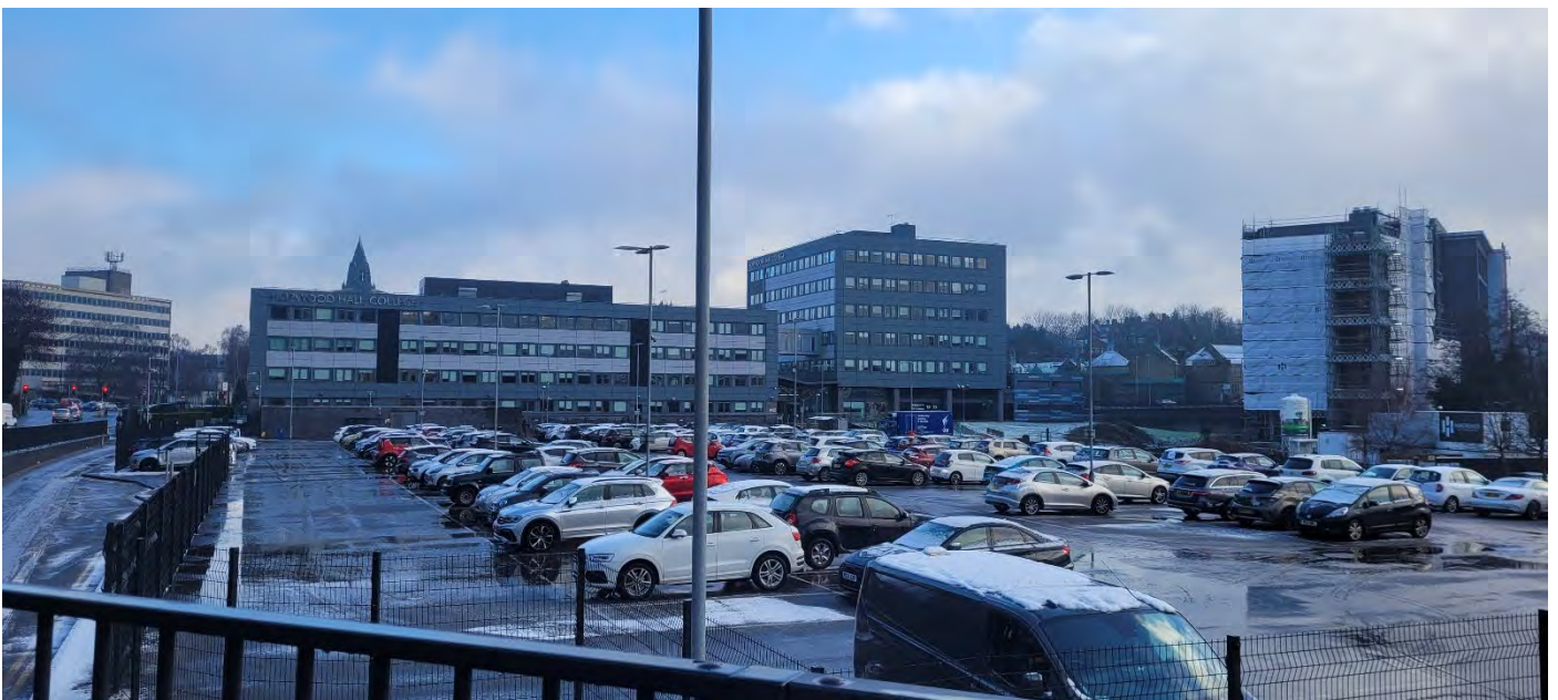
Plate 13 View of car park and Hopwood Hall College buildings, looking east
