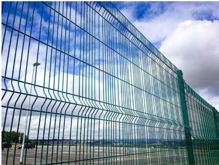
Typical Paladin fencing detail
