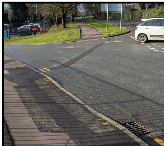
Picture 3-30 - Pedestrian Crossing Over Unadopted Access Road
