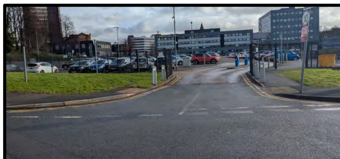
Picture 3-33 - Uncontrolled Pedestrian Crossing Over Hopwood Hall Car Park Vehicle Entrance
