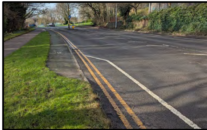
Picture 3-8 – Westbound Cycle Route Changing from On-Road to Off-Road Infrastructure
