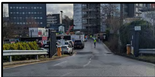
Picture 3-17 - Vehicle Access into Rochdale 6 th Form College
