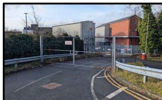
Picture 3-18 - Vehicle Access into Electricity Northwest Site
