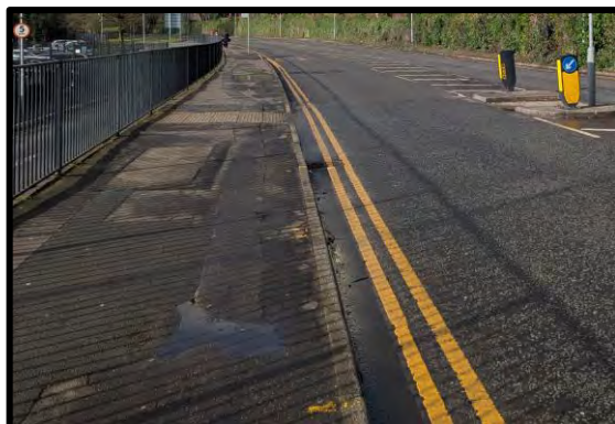
Picture 3-5 - TRO's in place on College Road
