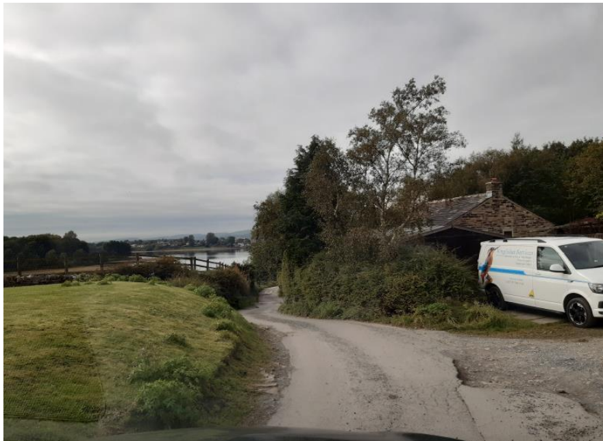
Figure 3 – View down Syke Road facing west, existing access on left.
