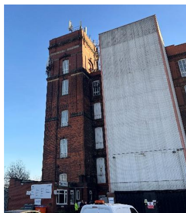
Fig 2.3 Tower to Northwestern corner.
