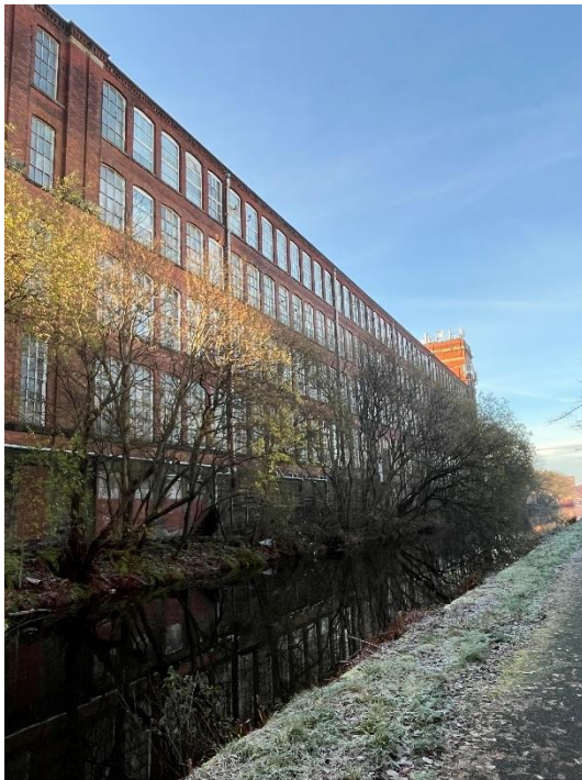
Fig 2.4 Rear of building along the canal
