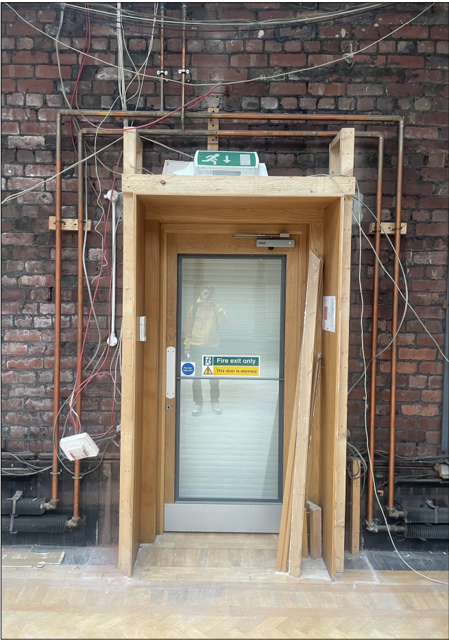
Image 01/04 - Example area around escape door where existing wall coverings have been removed (historically). The exposed brickwork was uncovered following the exhibition boards removal.
