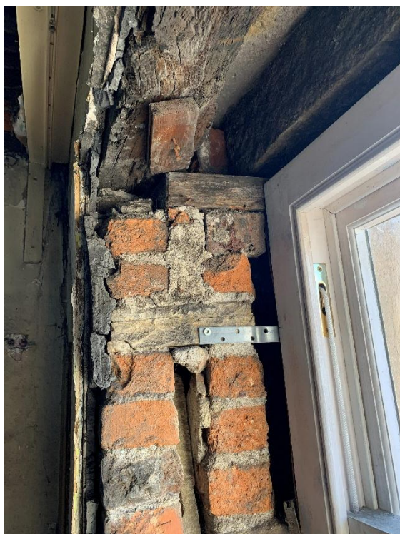
Figure 4.6: Window reveal in Room SF7.
