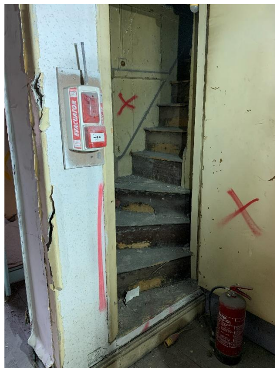
Figure 4.7: Dogleg stair in Room SF7
