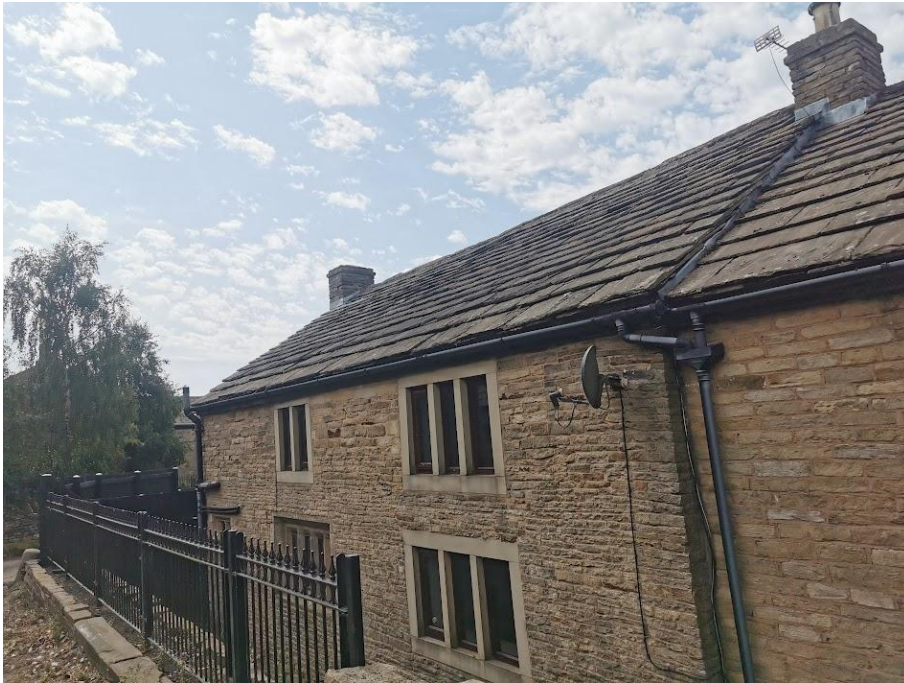
Photograph 1- Front (eastern) elevation of B1
