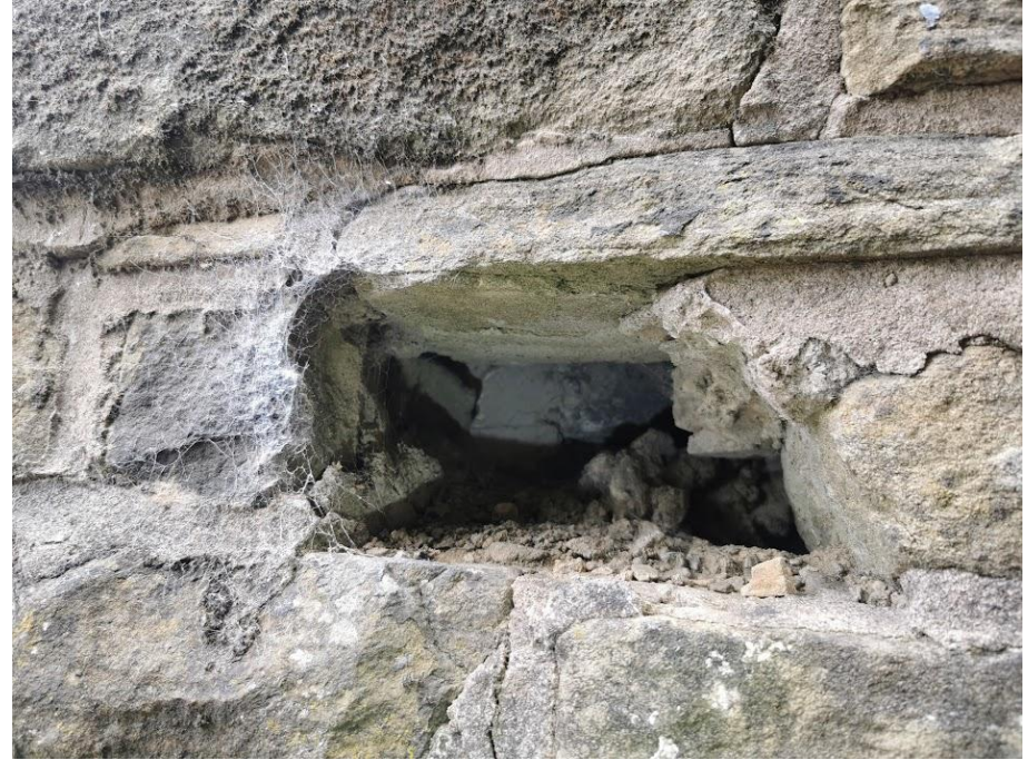
Photograph 12- Interior access point on southern elevation of B2
