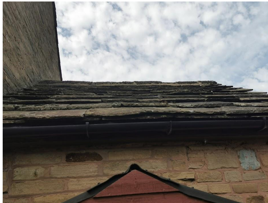
Photograph 6- B1, north eastern elevation
