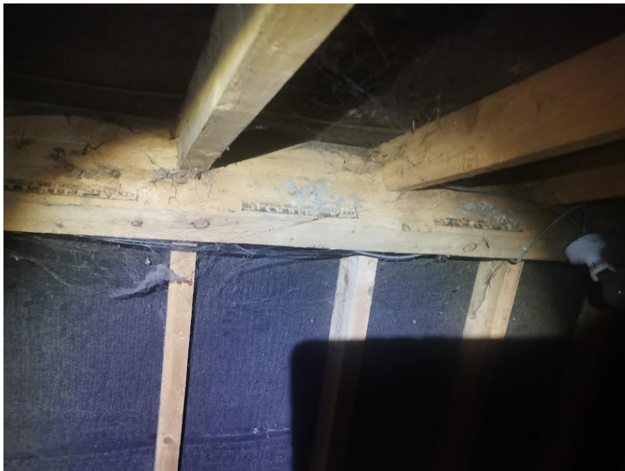
Photograph 5- Loft space of B1 showing cobwebs and well sealed
