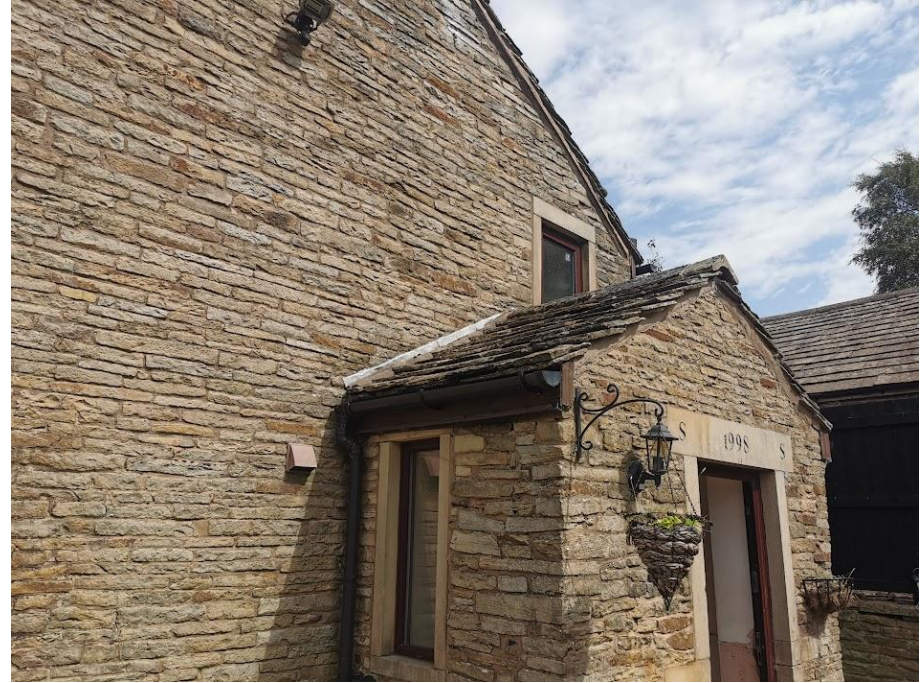
Photograph 4- South western elevation, porch area.
