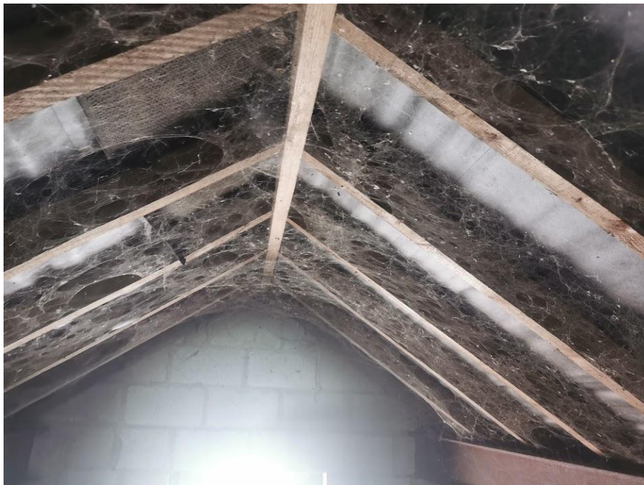
Photograph 9- Interior of B2 showing heavy cobwebbing
