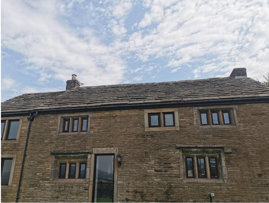
Photograph 3- Western elevation of B1.
