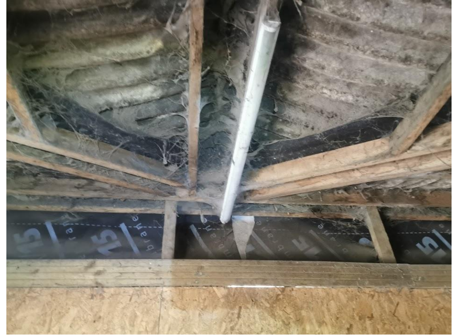
Photograph 14- Interior of B3 showing heavy cobwebbing
