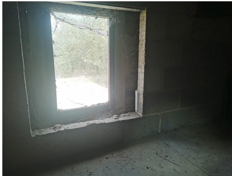
Photograph 10- Light ingress through windows into B2
